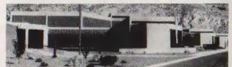
El Paso Gas Company Computer Center.
