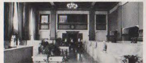
Old State Bank Building.
