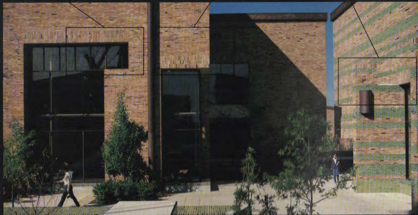
Punched keyhole fenestration within the Acme Brick bearing wall mirror the repetitive shapes of the cantilevered corner elements.
