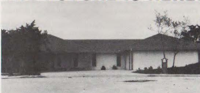
This 2900 sq. ft. San Antonio home is built of concrete block and SUREWALL® Surface Bonding Cement. Designer: Cardenas-Hardy and Associates.
