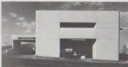
First City National Drive-in Facility.
