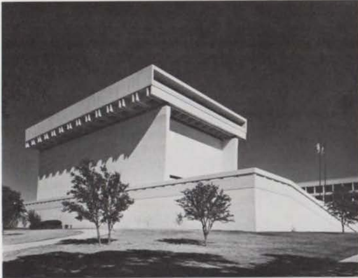
LBJ Library, Austin, 1971. Skidmore Owings and Merrill, Chicago. Brooks, Barr, Graeber and White, Austin (now 3D/International), associate architects.
