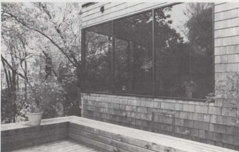
View toward living room and "bridge" wing from lower deck.
