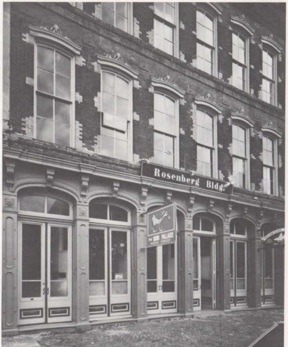
Strand-side facade, with all original ironwork restored.
