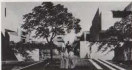
Junior college complex, Riyadh, Saudi Arabia, under construction. James M. Sink Associates, Houston.
