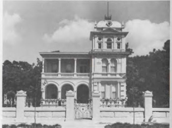
The Norton/Polk/Mathis House, King William Historic District, San Antonio, 1881. One of many in this district, which is undoubtedly "a superb collection of eclectic styles."—Sinclair Black, Austin.
