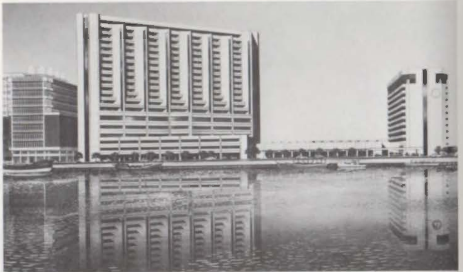
Inter-Continental Plaza, Dubai, United Arab Emirates, under construction. 3D/International, Houston.
