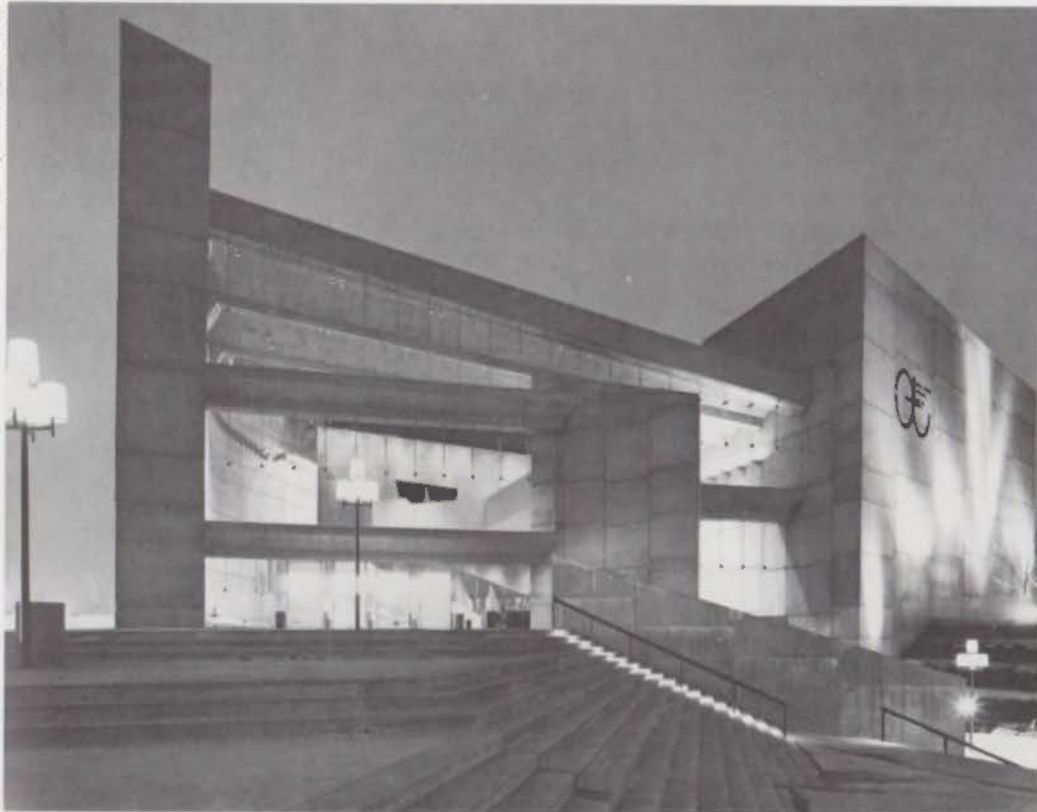
Edwin J. Thomas Performing Arts Hall, University of Akron, Akron, Ohio, 1973. Caudill Rowlett Scott, Houston. Dalton, Van Dijk, Johnson & Partners, Cleveland, associate architects.
