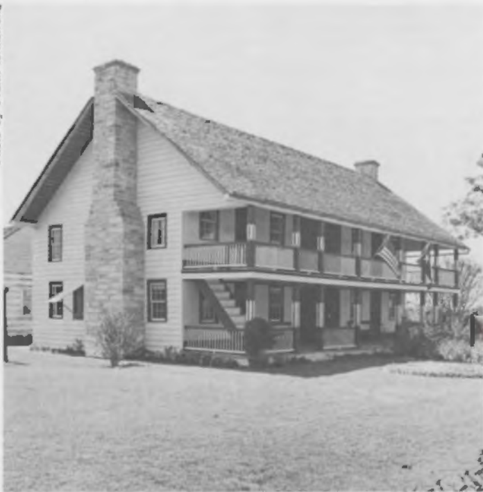
Sam Lewis House, Winedale museum complex, Round Top, 1848. Restoration begun 1961, Wayne Bell, architect.
