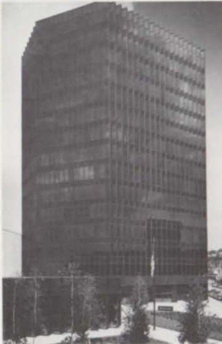
One Valley Square, Charleston, West Virginia, 1975. S. I. Morris Associates, Houston.
