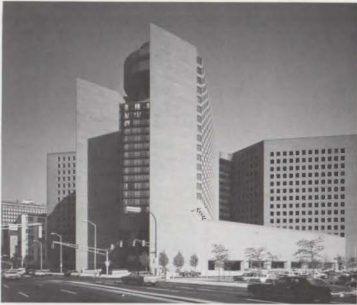
Merchants Plaza, Indianapolis, Indiana, 1977. JVIII Architects (Koetter Tharp Cowell & Bartlett, Caudill Rowlett Scott, 3D/International), Houston.
