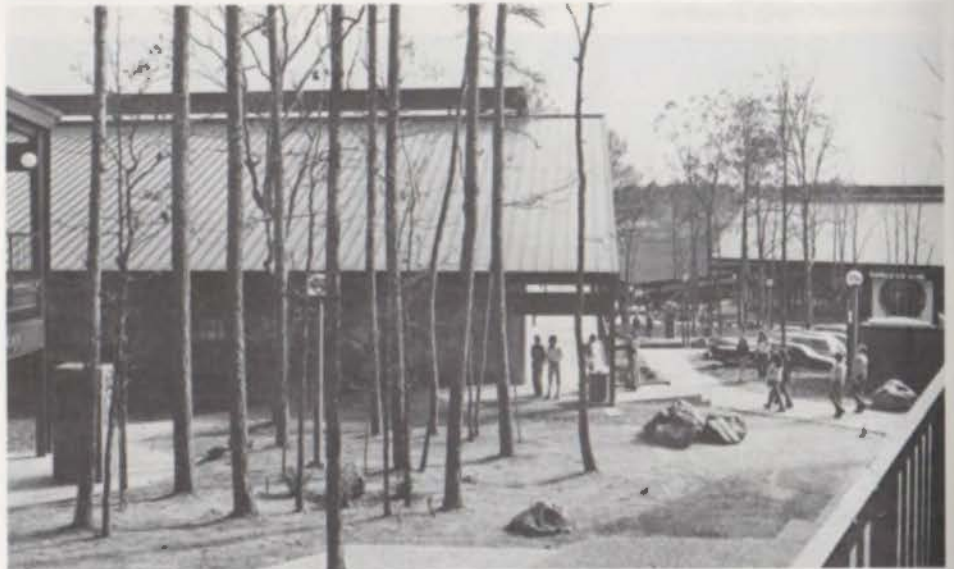
Breckenridge Village Shopping Center, Little Rock, Arkansas, 1976. ANPH, Dallas.
