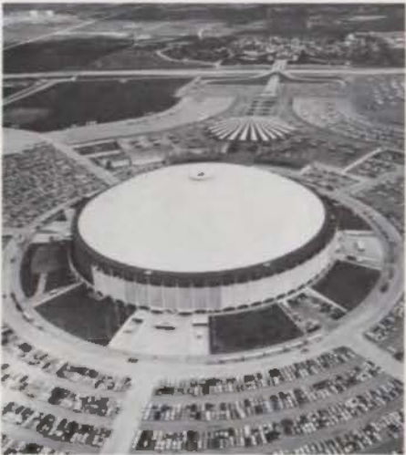
Astrodome, Houston, Lloyd & Morgan, and Wilson, Morris, Crain & Anderson, 1965. "Bold when it was built—the prototype for a generation of large indoor stadiums."—Jack Craycroft, Dallas.
