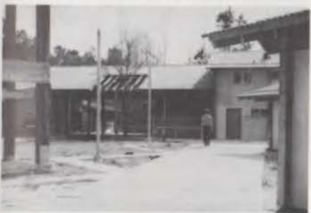
Three "H" Service Center, Houston.
