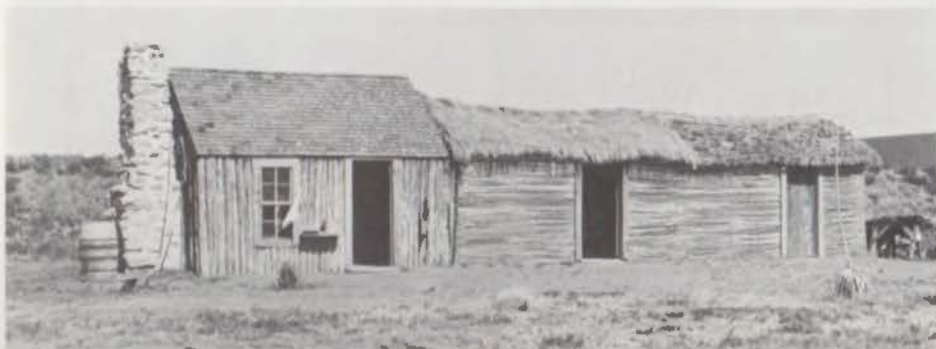
TOP, LEFT: Picket and Sotol House on original site. Note overgrowth, gaps in roof, pickets. LEFT: Picket and Sotol House after reconstruction. BELOW: Reconstructed interior of Sotol and Picket House.
