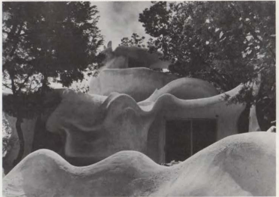
West facade; carefully planned view corridors.
