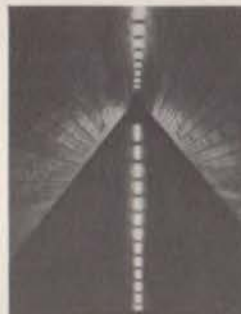
Heavy wood decking and continuous strip skylighting emphasize the exciting lines and soaring spaces of Grace United Presbyterian Church. The Greenville church is a Texas Architecture 1968 selection.
