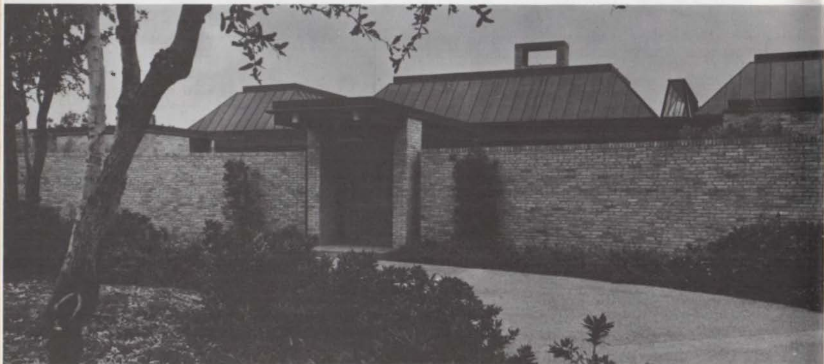
Sharp angles of roofs contrast with the curve of the wall and hard, straight lines. The ornate gates give an indication of the richness of the interior.
