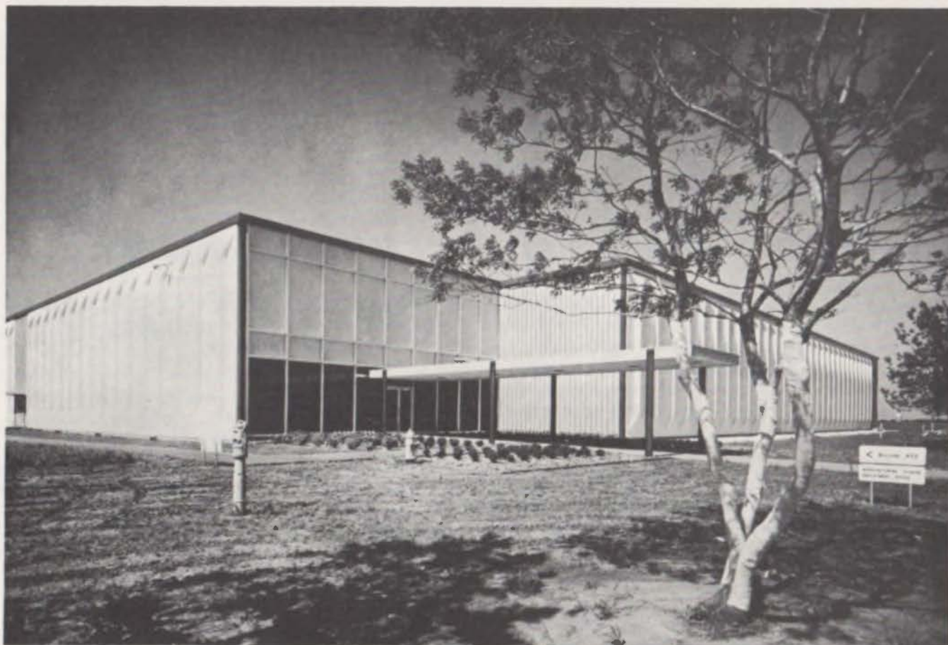
CREDITS: — Architectural & Engineering Div. of Collins Radio Co., Architect; A. C. Martin & Associates of Los Angeles, Architectural Consultant; Alpha of Texas, Inc., A Subsidiary of Collins, General Contractor; McDonald Brothers Cast Stone Company, Fort Worth, Texas; Gregerson & Guyour, Inc. of Dallas, Mechanical-Electrical Engineers, and Mullen & Powell of Dallas, Structural Engineers.
