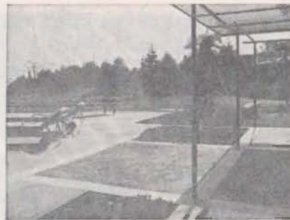
Terraces built of contrasting exposed aggregate squares are striking sales-winners.
