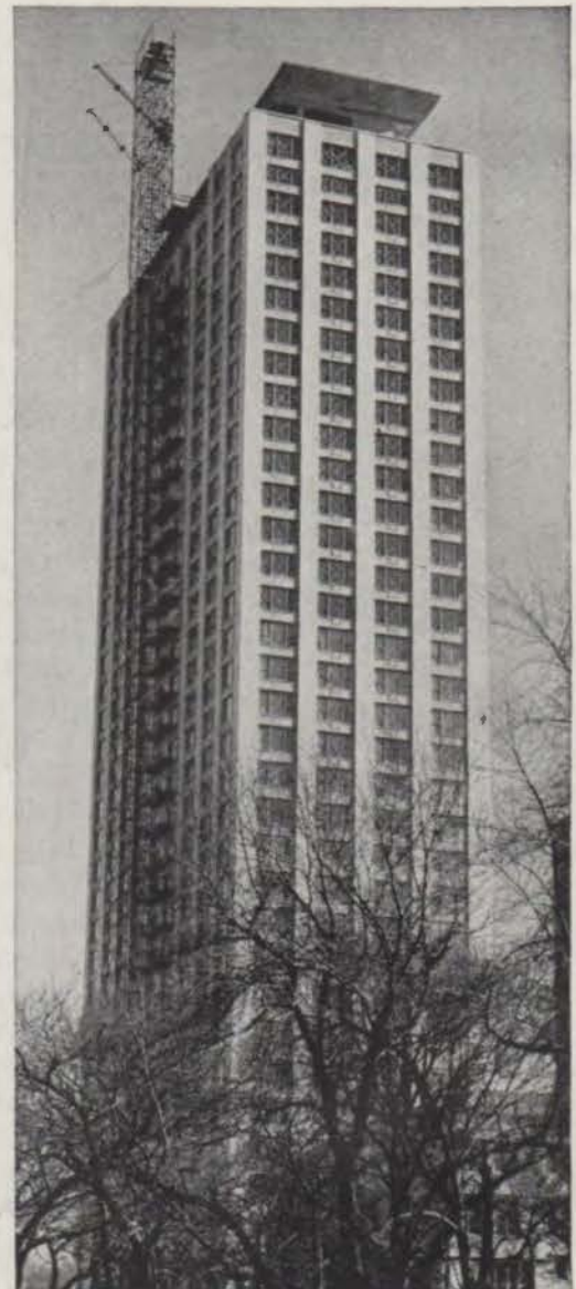
Here, the 35-story apartment building nears completion
