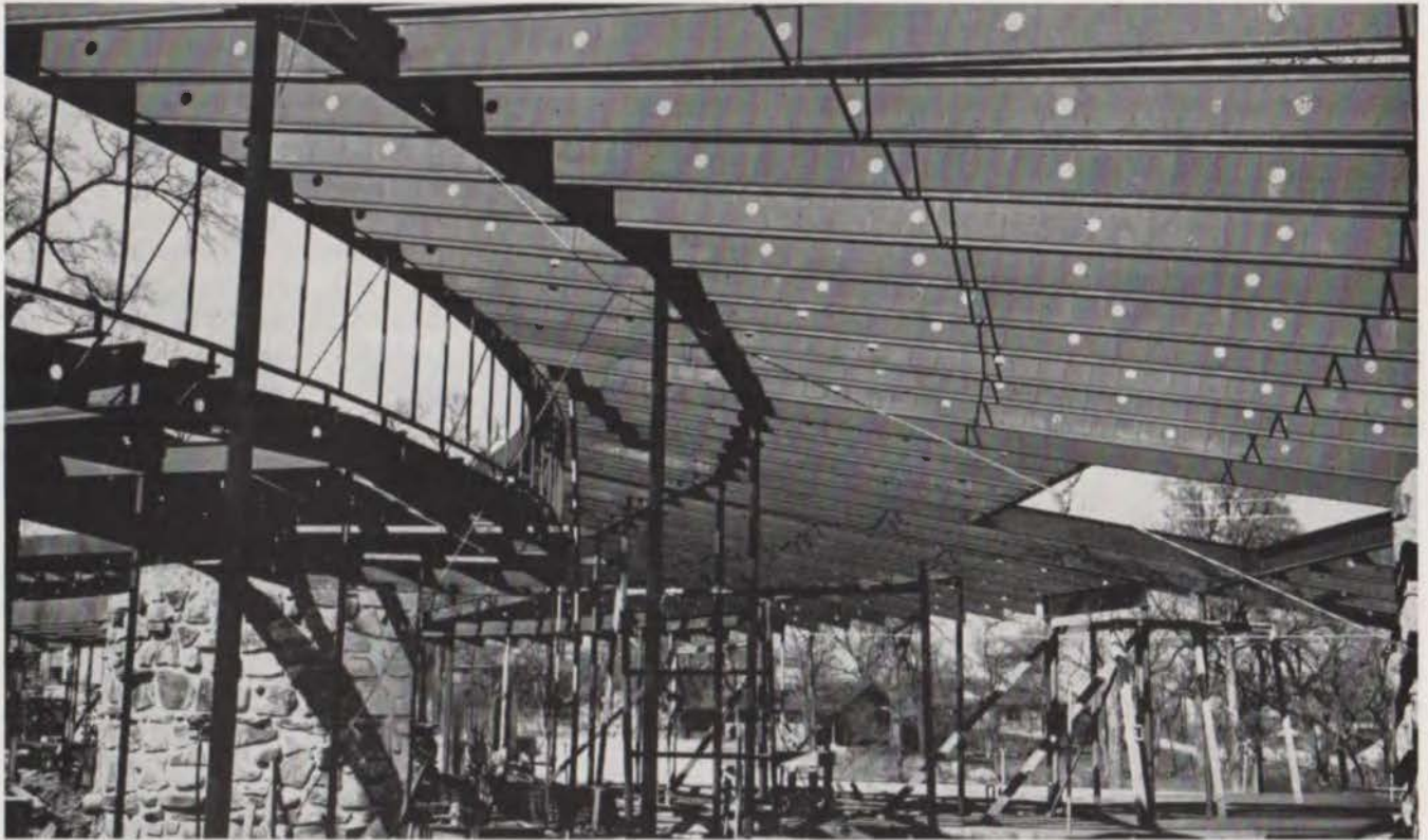
Stran-Steel joists form semi-circular roof and terrace.
