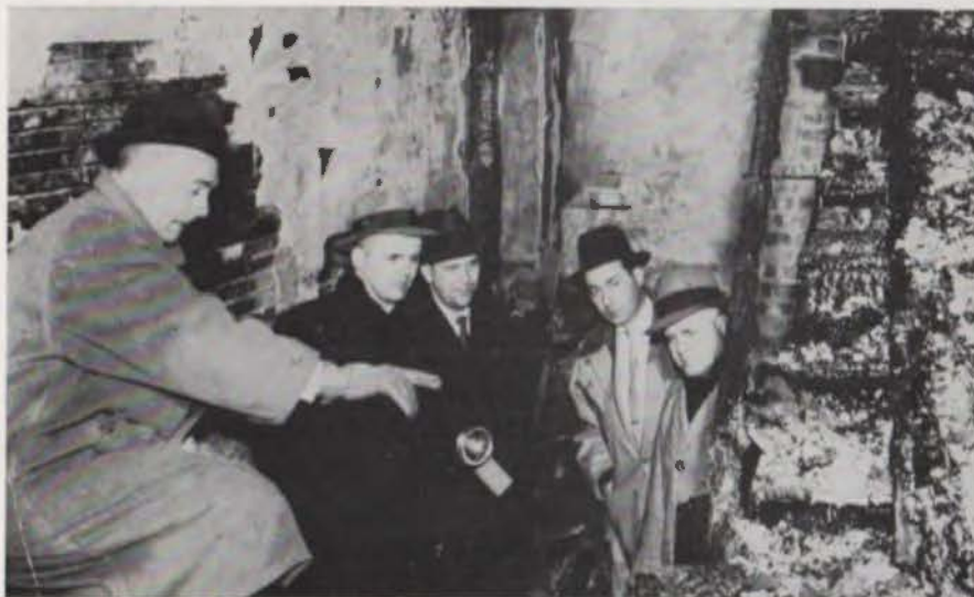
Officials of the Chicago Police Department and Coroner's Office examine the stairwell in which the tragic school fire may have started. (Photo courtesy of "The New World.")
