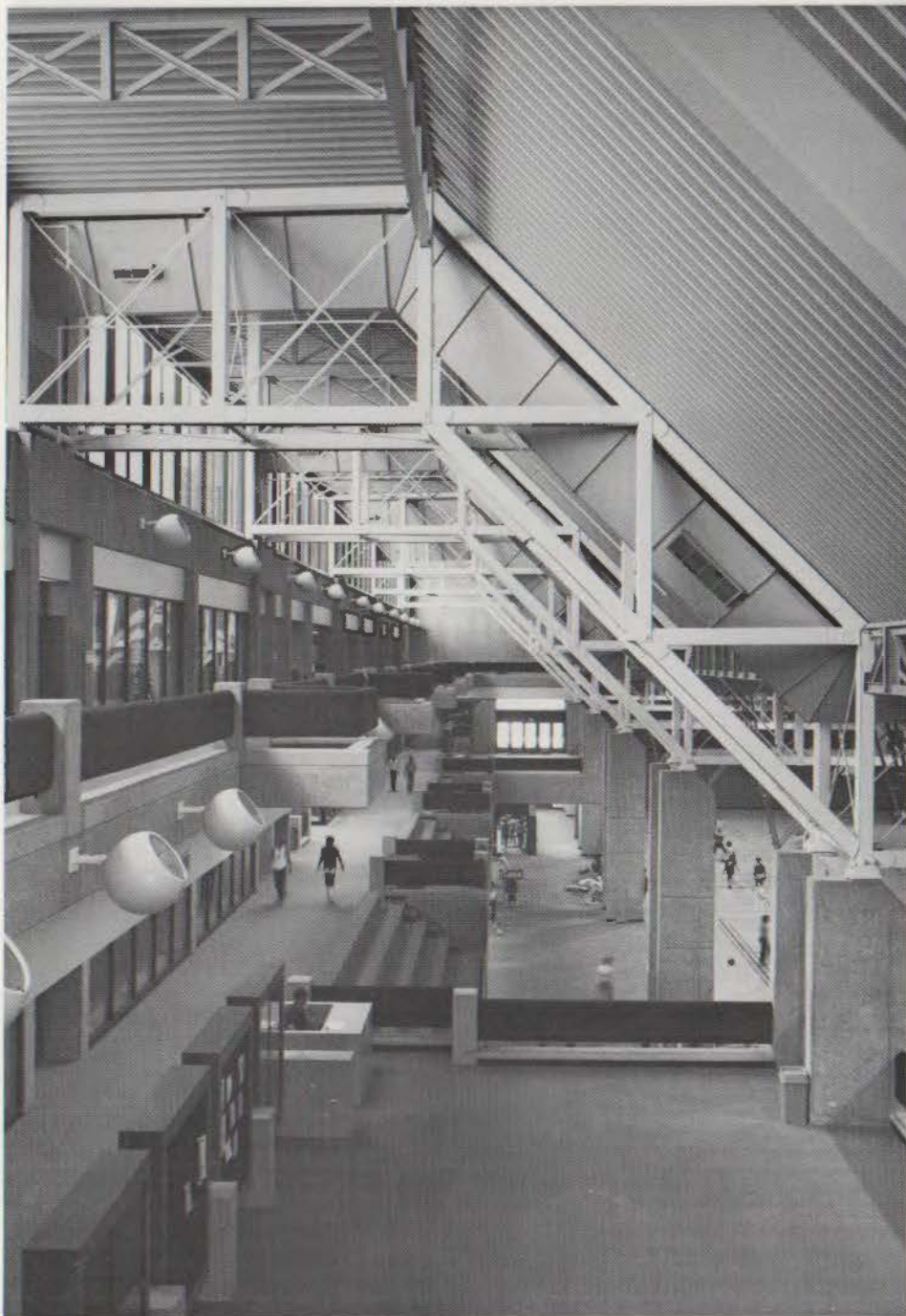
Trusses rising above second and third level overlooks.
