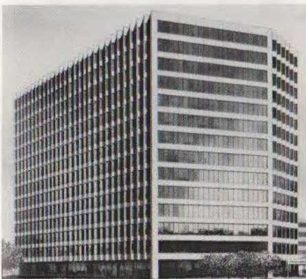
Midland National Bank Tower II, Midland, for Gerald D. Hines Interests, Houston. Building architects: Morris * Aubry Architects, Houston.
