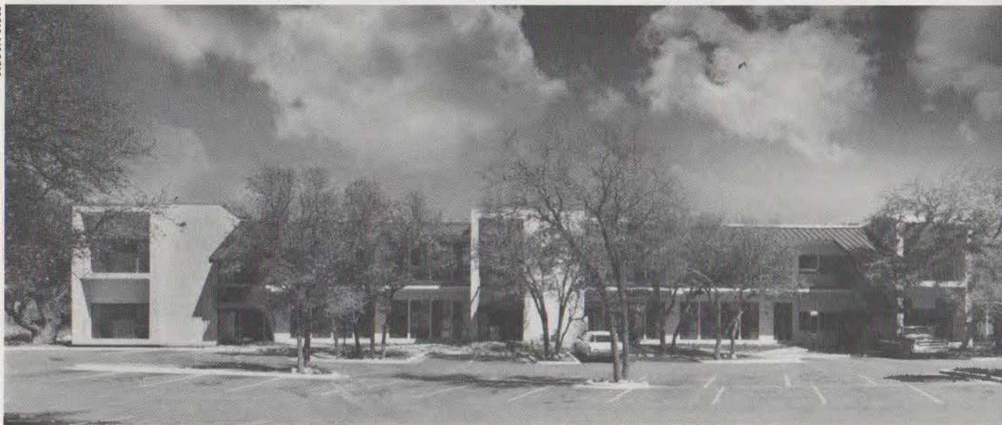
Passive-solar commercial building in Austin.
