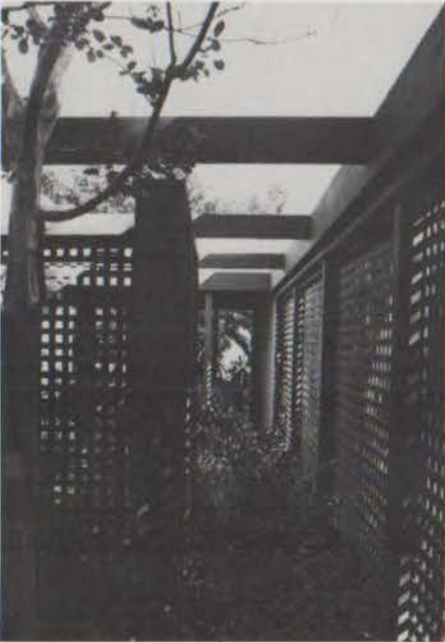
Trellis court extends interiors.
