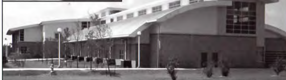
BERRIDGE LICENSEE PORT ENTERPRISES OF AUSTIN, TX, INSTALLED BERRIDGE CURVED HIGH SEAM TEE-PANEL FOR THE ROOF OF PALO ALTO COMMUNITY COLLEGE IN SAN ANTONIO, TEXAS.
