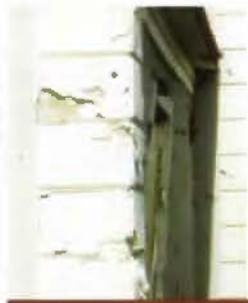
EIFS heavily damaged by high winds in Memphis.
