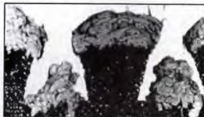
The Mortar Net holding mortar droppings from 32 courses of brick (8" wall).
