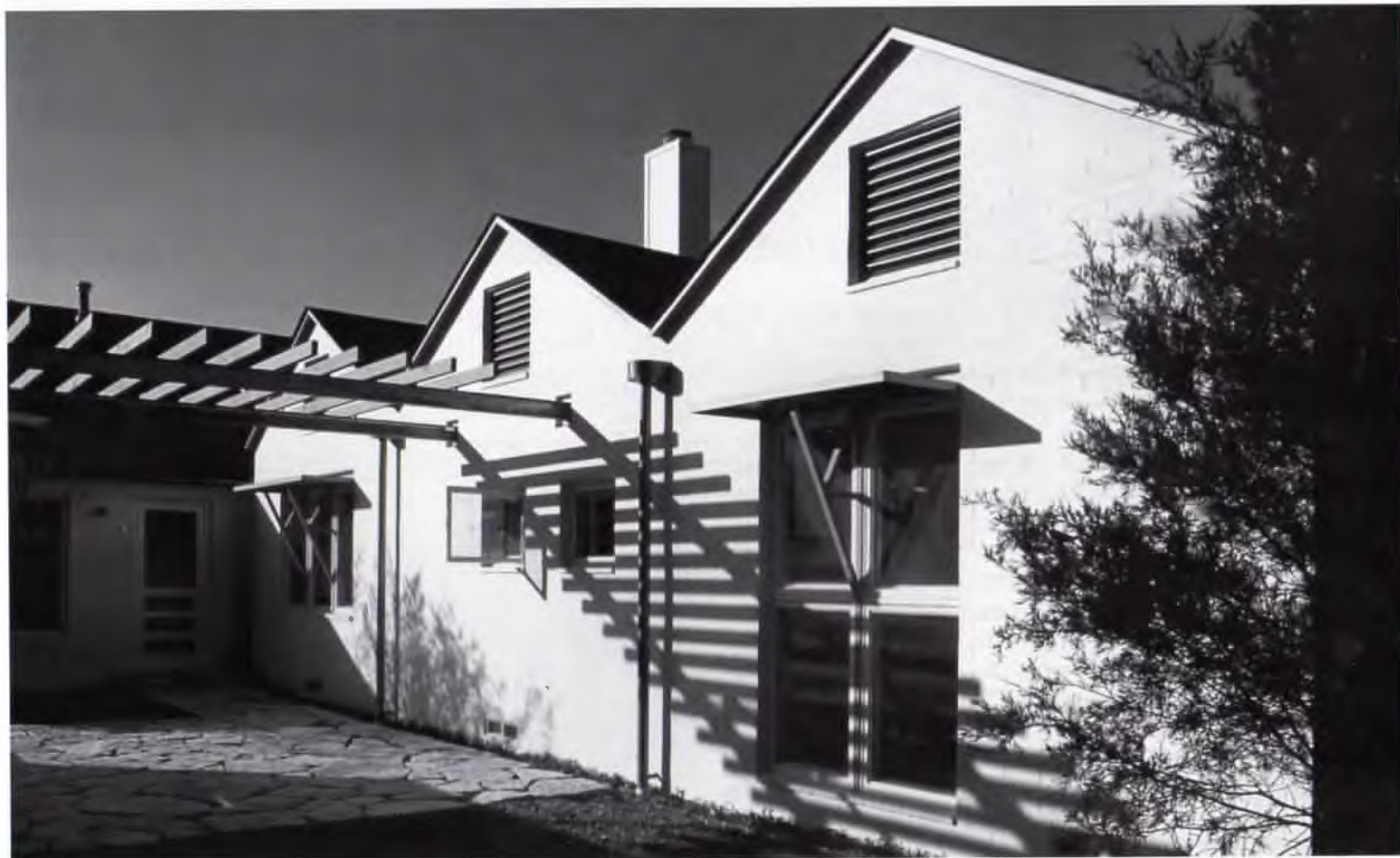
Below: the addition attached to the rear of the house
