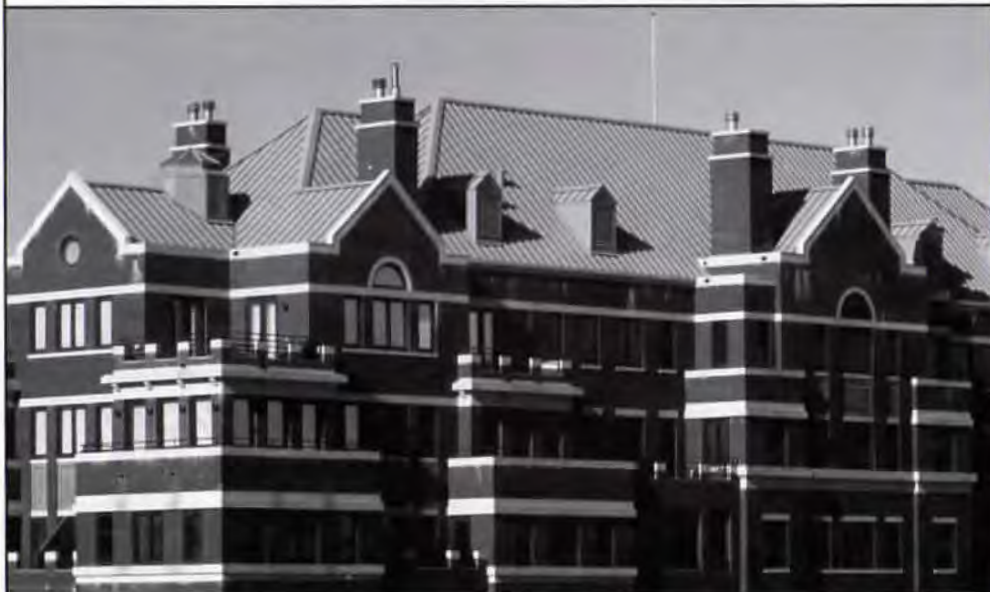
THE BOLD LINES OF BERRIDGE'S TWO INCH HIGH SEAM TEE-PANEL IN ARCADIA GREEN PROVIDES A FUNCTIONAL DESIGN STATEMENT ATOP THE SUNDANCE HIGH RISE APARTMENTS.
