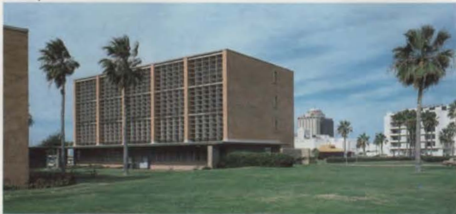
Richard Colley's now-vacant 1952 Corpus Christi City Hall may be razed to create bayfront park space.
