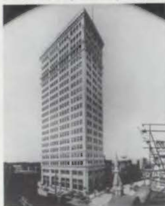
Amicable Building, Waco
