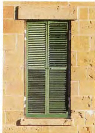
Window detail, Commanding Officer's Quarters
