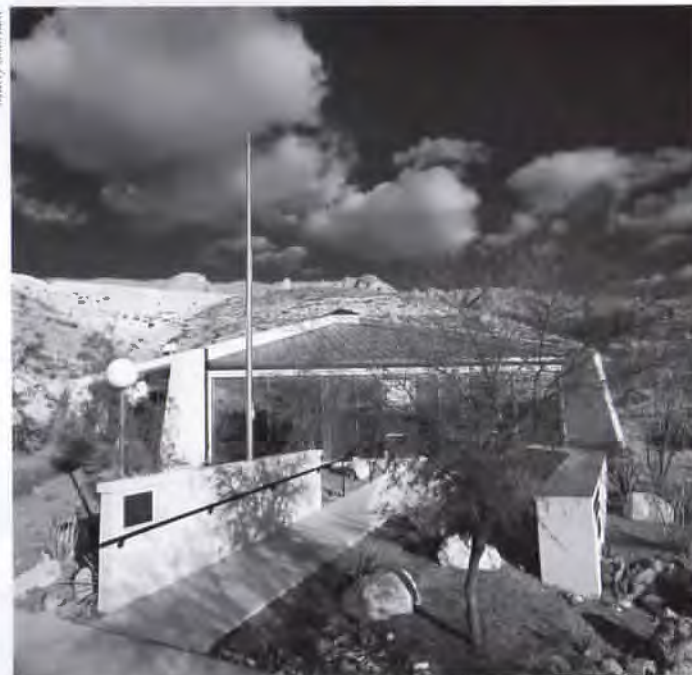
The American Heart Association building, by Edward E. McCormick (now a principal with McCormick, Kuykendall, McCombs, Suerken Architecture, Inc.) is a hexagonal glass-walled building hugging a dry hillside.
