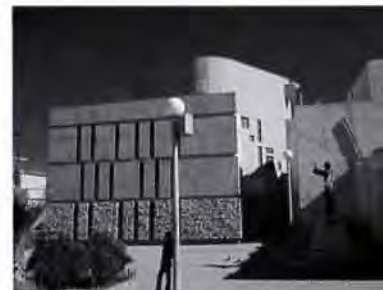
TOP: Grated light wells illuminate cathedral offices under the plaza. BOTTOM: Rear elevation of cathedral shows Corbusian forms and materials.
