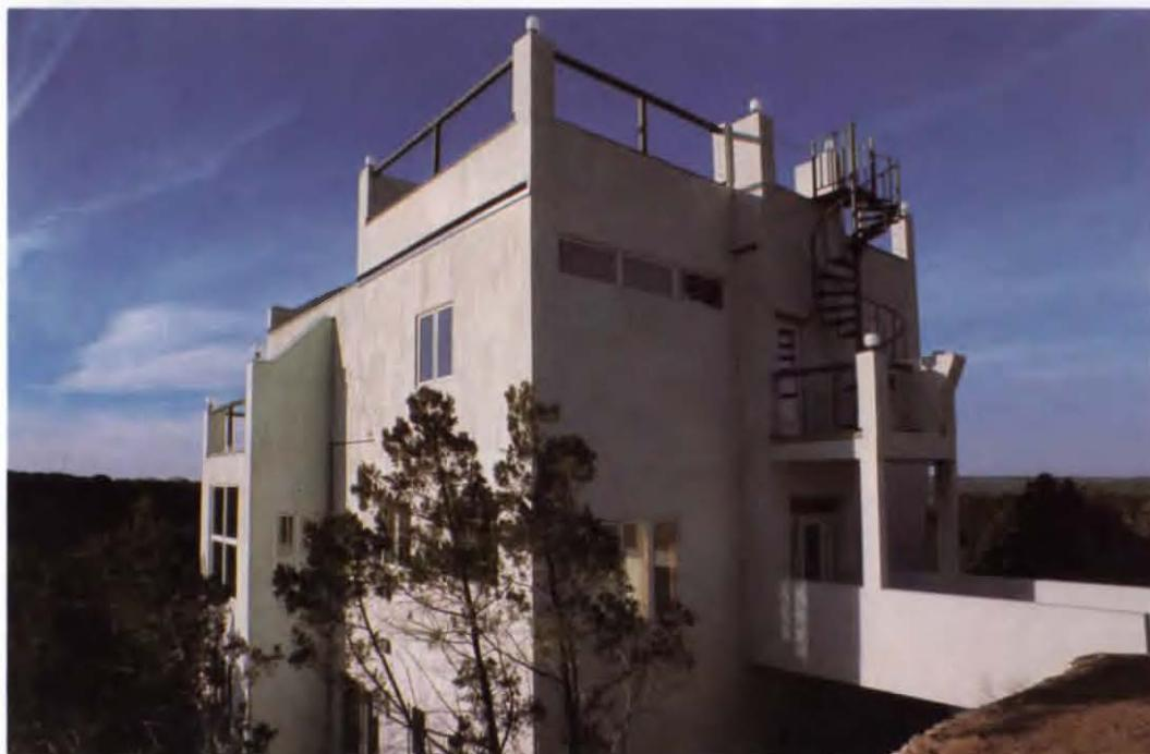
Southeast elevation: exaggerated keystone above entry-way catwalk fronts spiral stairs from bedroom to roof deck.
