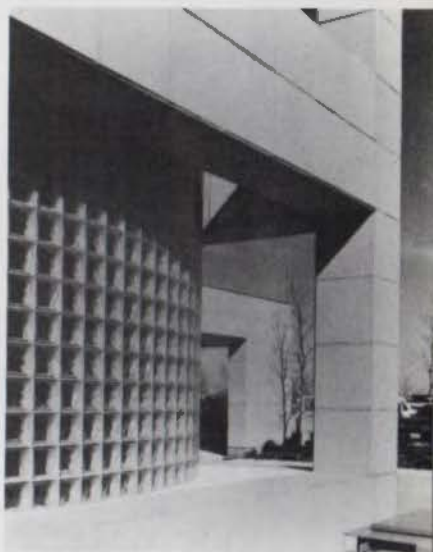
ABOVE: Walls of glass block surround curving stair enclosures. LEFT: The terminal's nighttime image is enlivened by the glow radiating from glass block openings.
