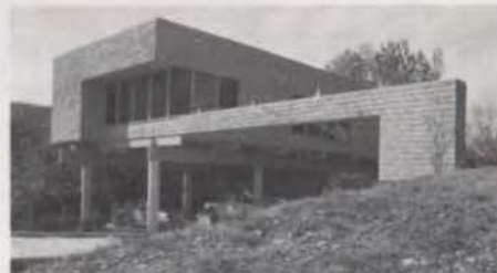
Vickery Creek Offices, Fort Worth
