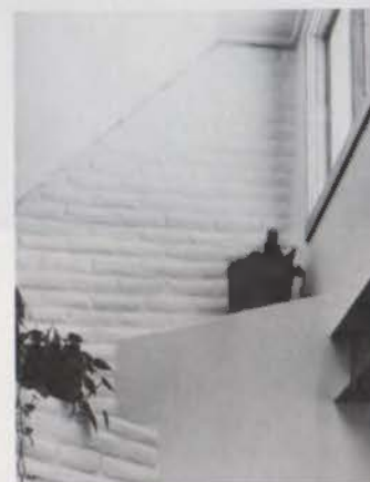
TOP: Pipe columns and beams are painted a vibrant blue to match the color of the El Paso sky. ABOVE: The intersection of two conference rooms forms triangular niches used as plant shelves.
