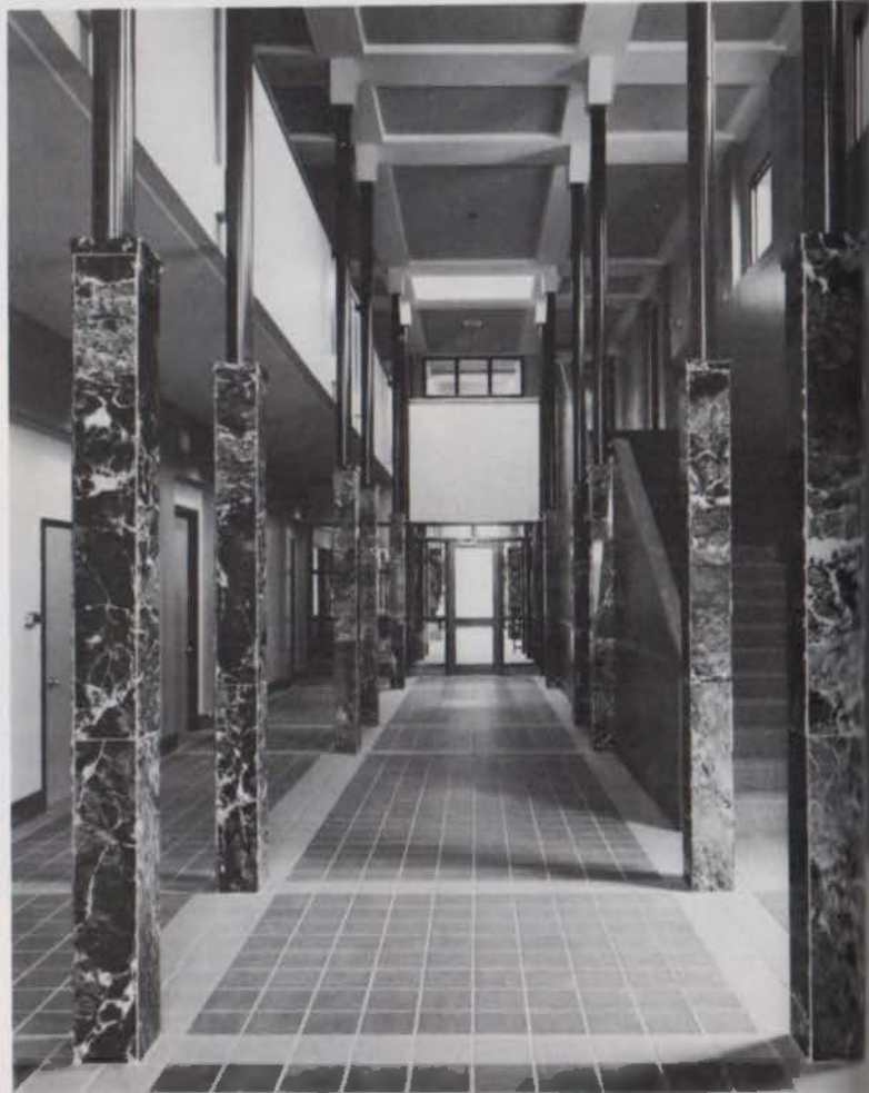
Marble-clad steel columns define double-height corridor leading through lease space to main lobby.
