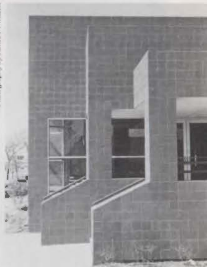
Because of its ability to cover disparate surfaces evenly, tile veneer was used to renovate this 1960s brick office/warehouse.
