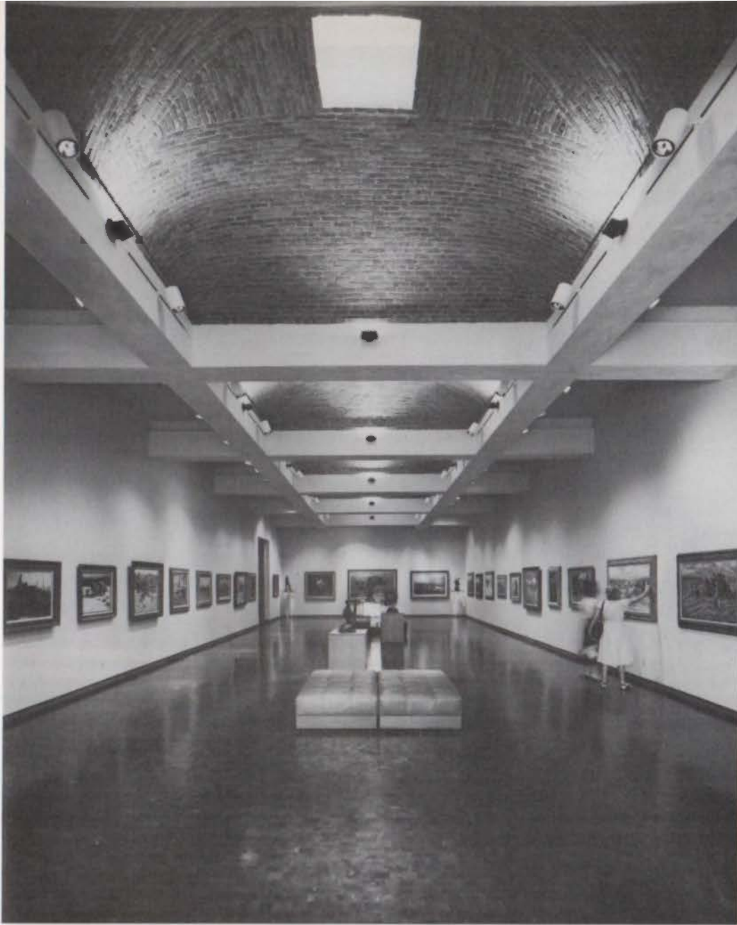
Brick bovedo domes, a Ford trademark, span the central 20 feet of the gallery, admitting light to the center of the room.
