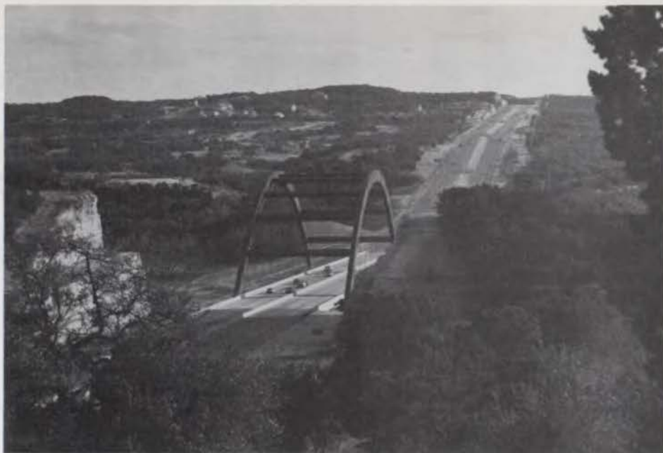
Loop 360 bridge spanning Lake Austin.
