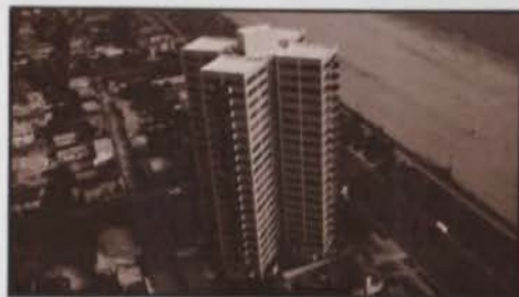
Galaxy Towers — on the Pacific at Long Beach — with roofs protected by Brai.
