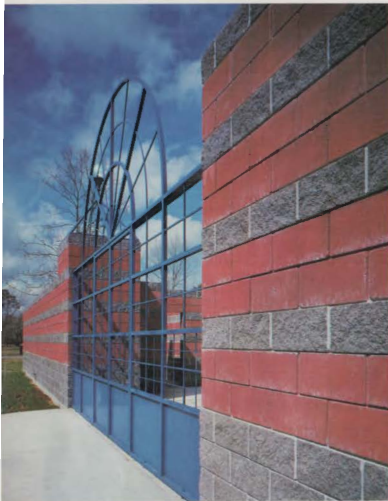
Walls are composed of concrete blocks—split-face grey and contrasting bands of smooth red.
