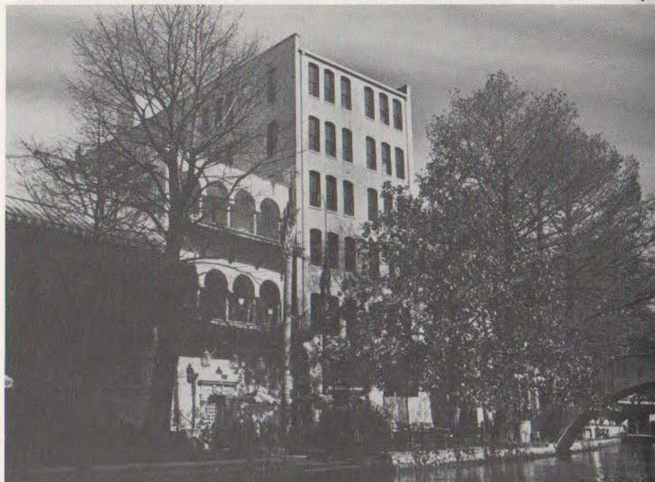
The old six-story Paseo hotel on the River Walk in San Antonio, soon to be the Lasoya.
