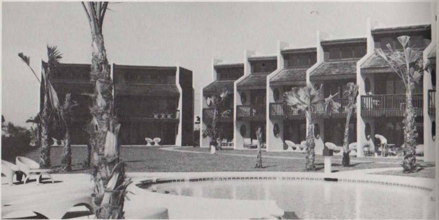
Suntides I, a 30-unit condominium complex on South Padre Island, Texas, was built of concrete blocks and SUREWALL® Surface Bonding Cement to withstand high velocity winds from the Gulf of Mexico. Architect on the project was Rick Labunski. General Contractor: Popkin-Williams Construction Co.
