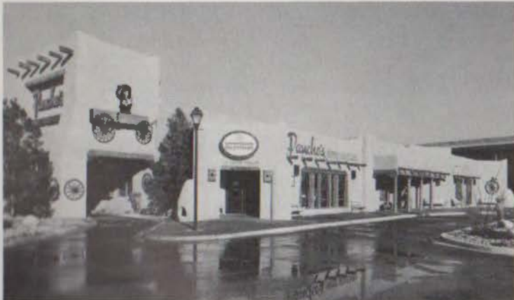
Surface bonded walls in a sand color create an adobe effect, yet are stronger and more durable, in the Pueblo Plaza Shopping Center, Las Cruces, New Mexico. Architect: Gerald Lundeen. General Contractor: Highland Enterprises.
