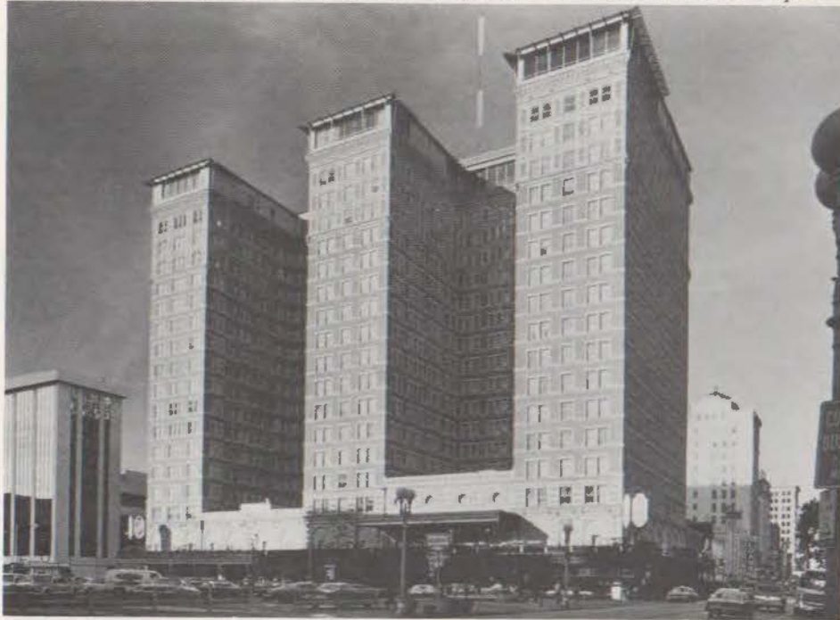
LEFT: Fox-Jacobs site in Dallas. BELOW: Houston's Rice Hotel and Lovett Square.
