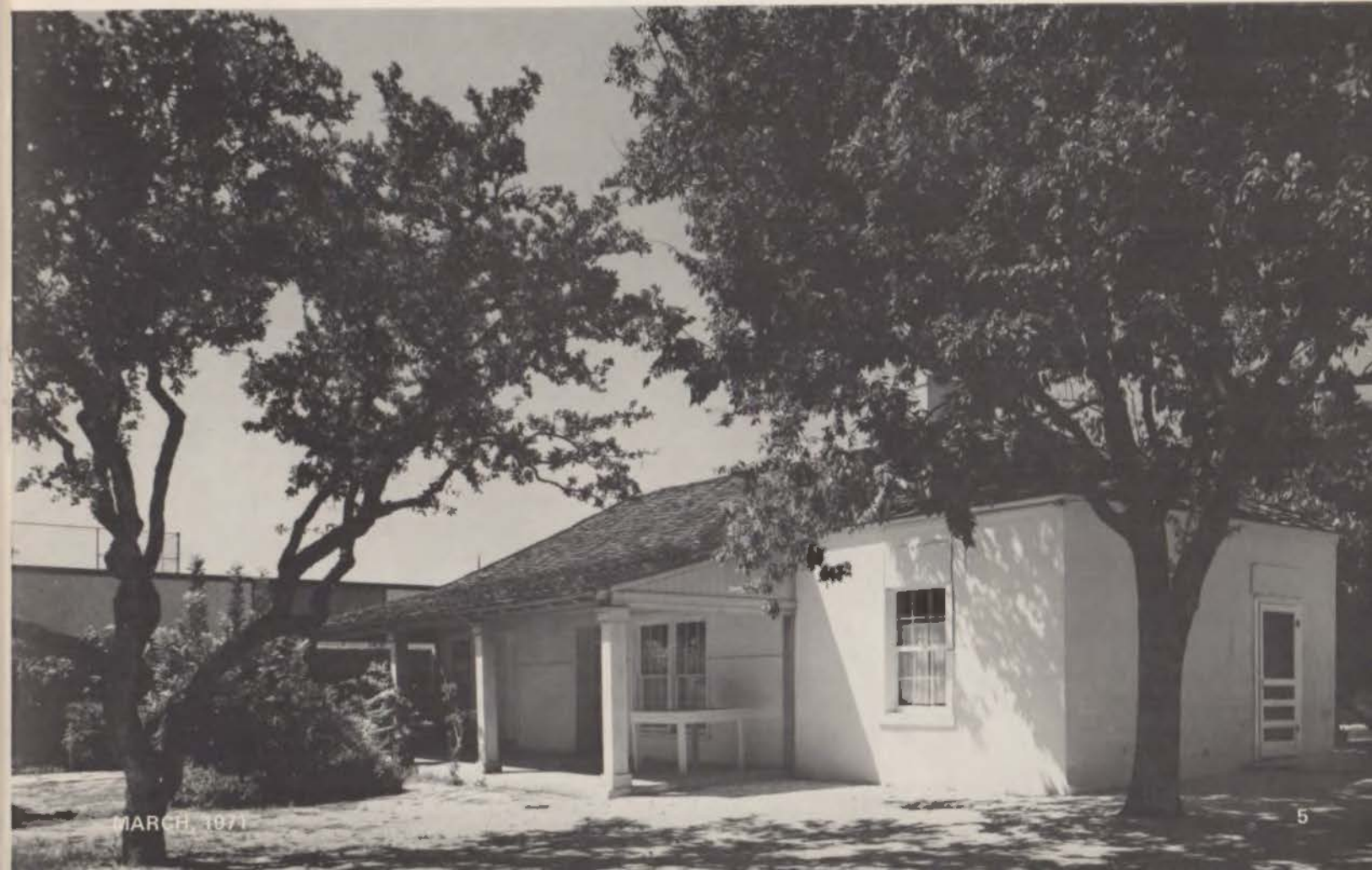
view of kitchen from rear
