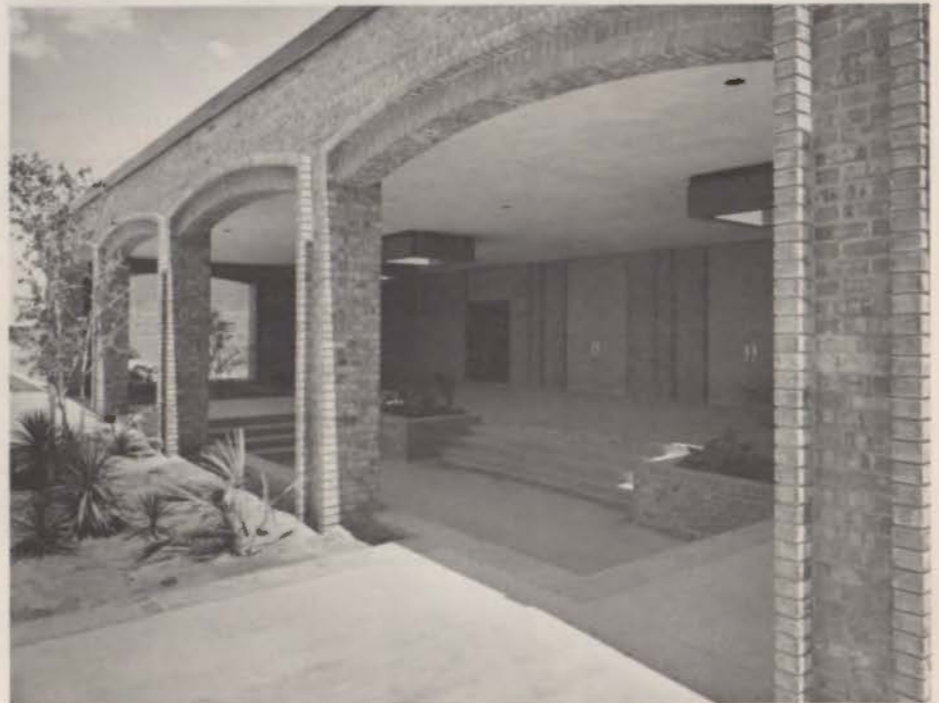
main entrance thru learning court
