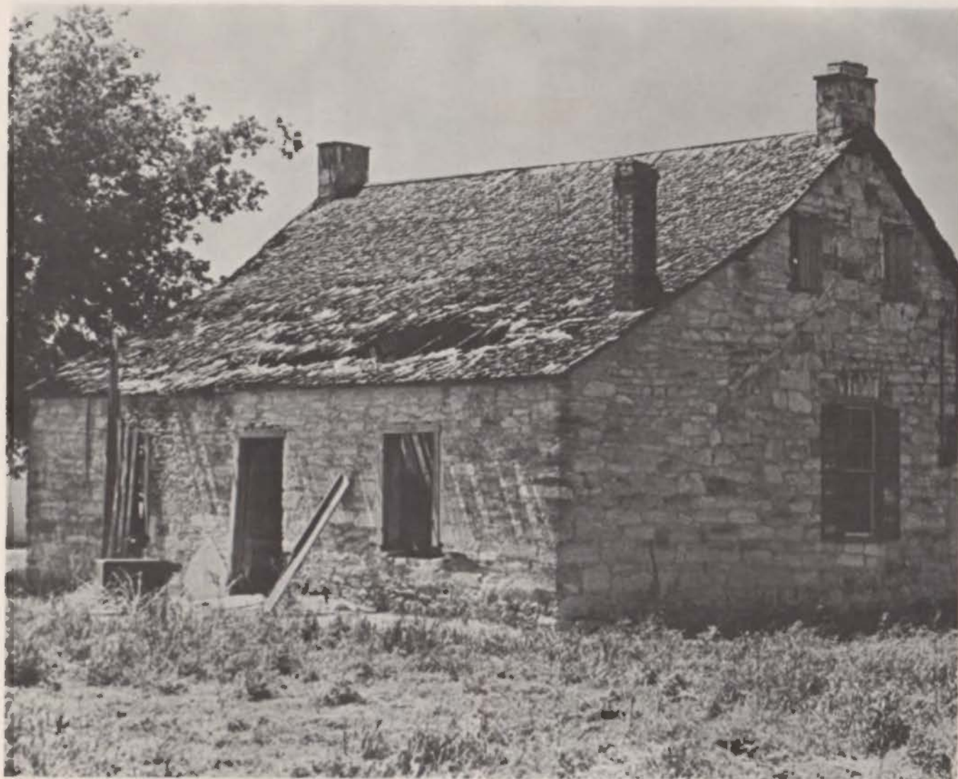
HALLER HOUSE, CASTROVILLE — NOTE CHIMNEY OVER FIRST FLOOR WINDOW
