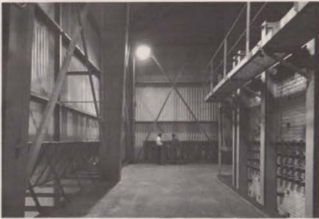
View of furnace building showing a portion of the regenerator-furnace on the right and adjustable vents to the left and rear through which air is pulled to cool both the furnace and personnel.
