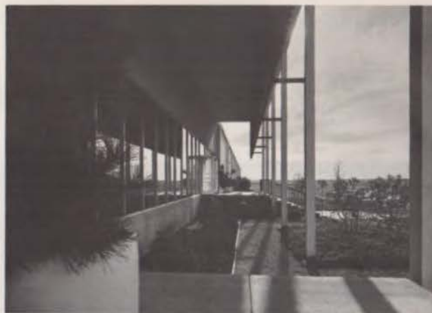
View of main entrance porch with employee entrance in the background.
