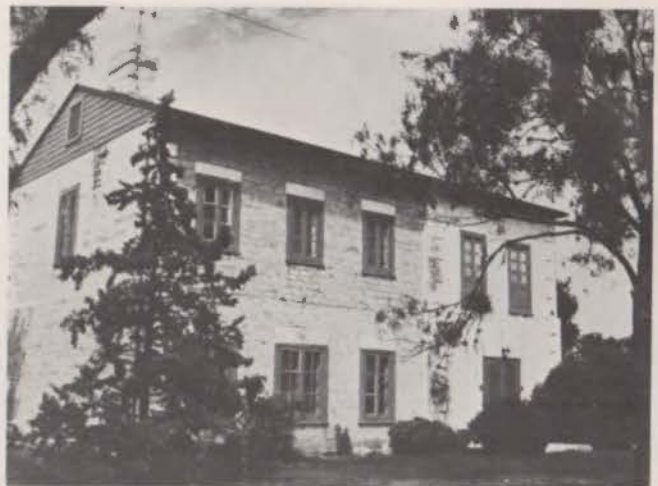
METZGER HOUSE, NEW FOUNTAIN STONE BARN, NEW FOUNTAIN
