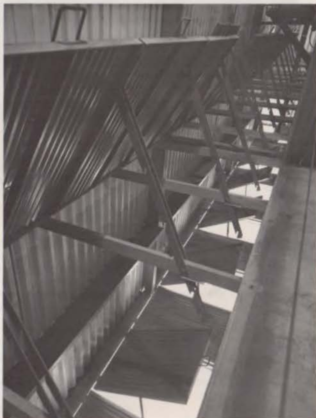
Detail of adjustable vents around furnace building. Air is pulled from exterior and the volume controlled by these vents.
