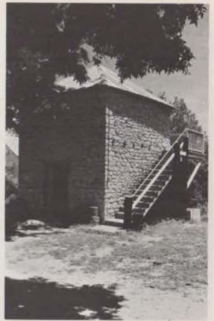
VANCE BATHHOUSE, CASTROVILLE
