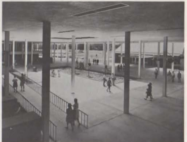
Spring Woods High School is spacious building with all classrooms reached from mall area. Wheel chair ramp at lower left and auditorium entrance is at right.
