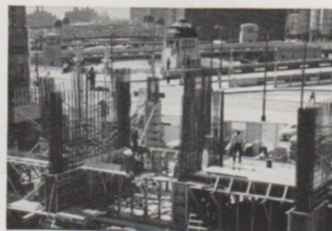
Four concrete shear walls extending across the width of the building provide necessary resistance to wind forces.
