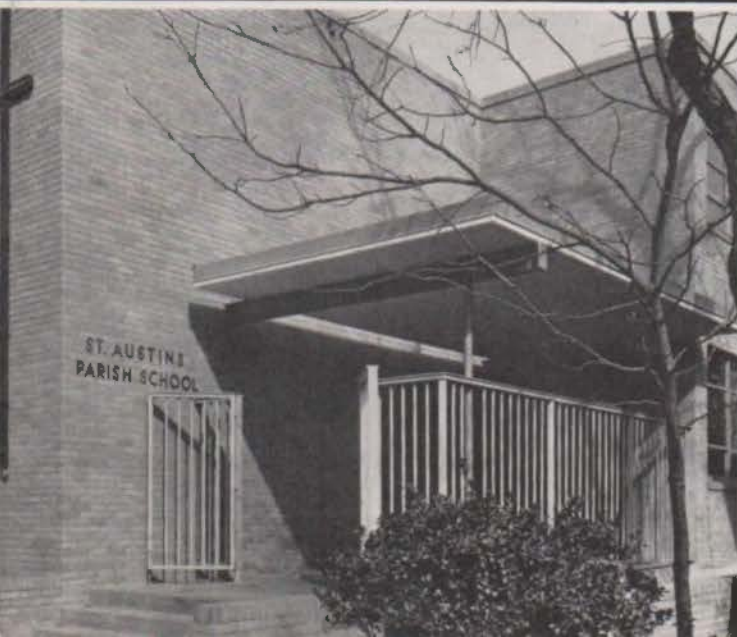
Front entrance of St. Austin's Parish School, Austin, selected by the Central Texas Chapter, TSA-AIA as representative of recent work in the Chapter area. Architects: Page, Southerland & Page, TSA-AIA, Austin.
