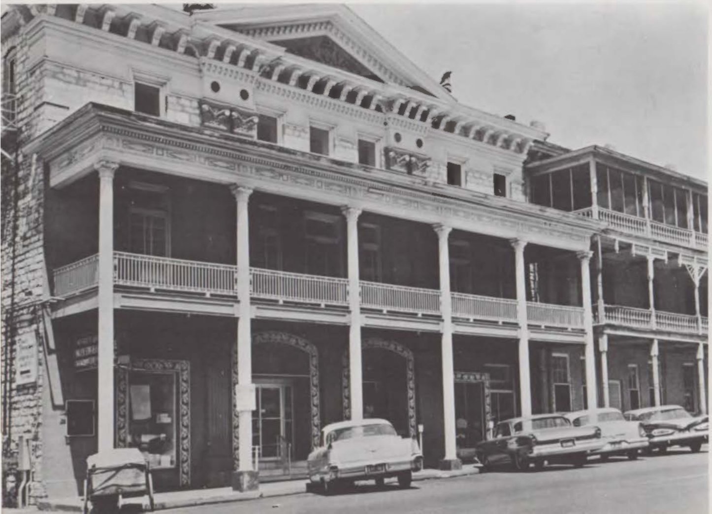
New Facade Added in 1911
