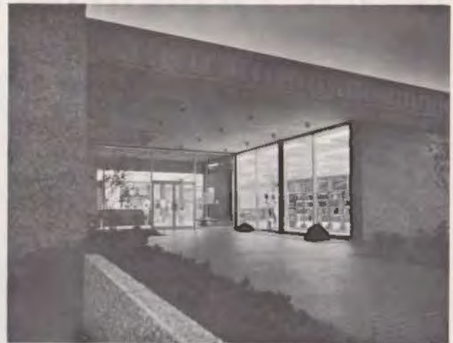
Dallas Public Library, Casa View Branch Wm. H. Hiddell, A.I.A. Architect
