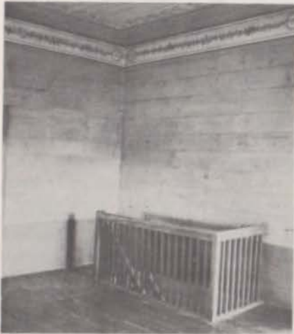
Stair confined to corner with awkward rise and tread dimensions.
