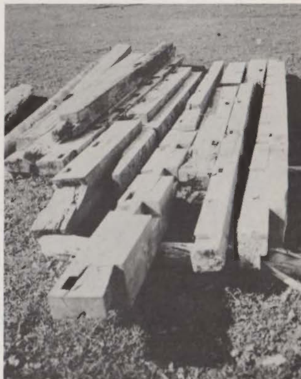
Notched members from a barn.
