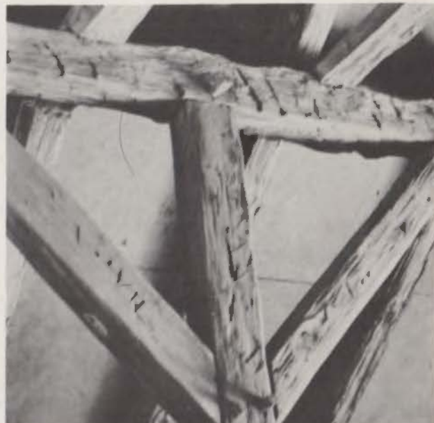
Hand hewn structural members from large barn. Note Roman numerals and wood pegs.
