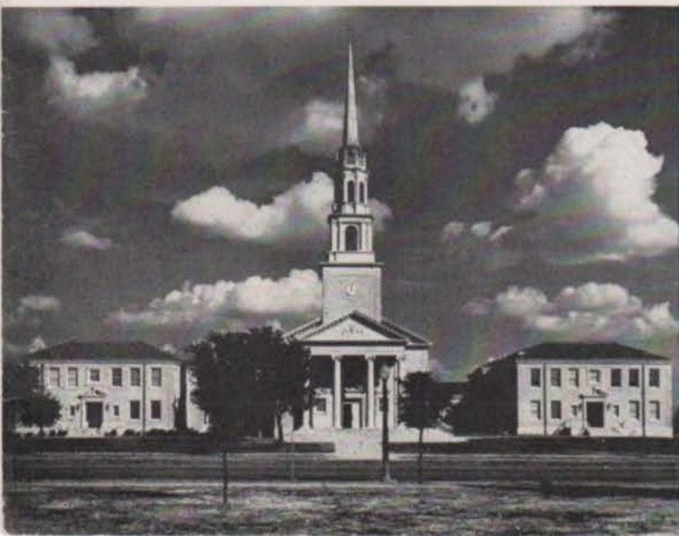
Robert Carr Chapel at Texas Christian University has been selected by the Fort Worth Chapter, AIA, as representative of recent work in the Chapter area. Architect: Joseph R. Pelich, Fort Worth.
