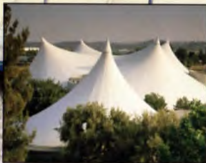
Over two decades of service in southern California.
