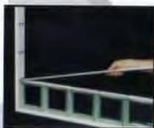
course. Next, the horizontal separator is laid on the blocks, extending from slot to slot at the sides. More than a spacer, the metal separator functions as a stiffener in every horizontal joint.
