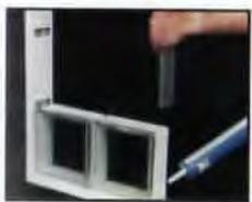
**1** Glass block sealant is applied to the center seam of the vertical edge of the block.
