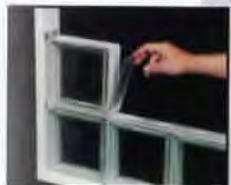
**3** Sealant is applied to the center of the horizontal separator and on the sides of
