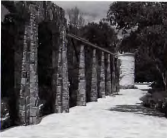
Left: Masonry arches carry water in a trough to the entrance cistern.
