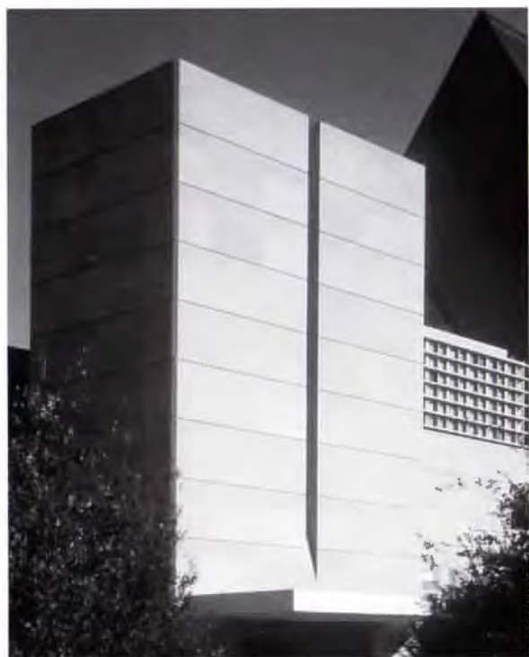
A "fortification tower" marks the north-side entry of the DMA's Nancy and Jake Hamon building, set in a skillfully planned vehicular court.
