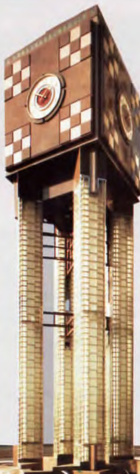
First Union Clock Tower Charlotte, NC Architect: JPJ Architects ARGUS® Pattern with Fibrous Glass Inserts HEDRON® I Corner Block, VUE® Pattern
