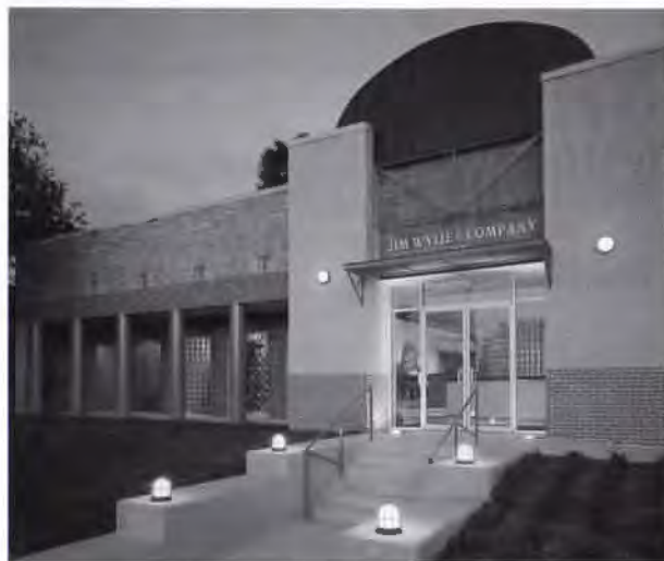
ABOVE LEFT: Jacob S. Anderson's 1955 Decorative Center, the first project in the Dallas Market Center, is a superb and original response to climate and program. The Contract Design Center, by WZMH Group. ABOVE RIGHT, and The Wylie and Co. showroom, designed by Sullivan Key Merrill. LEFT, are part of the Design District, an area of low-scale remodeled warehouses interrelated by lively design—the effect is something like a postmodernist costume party.
