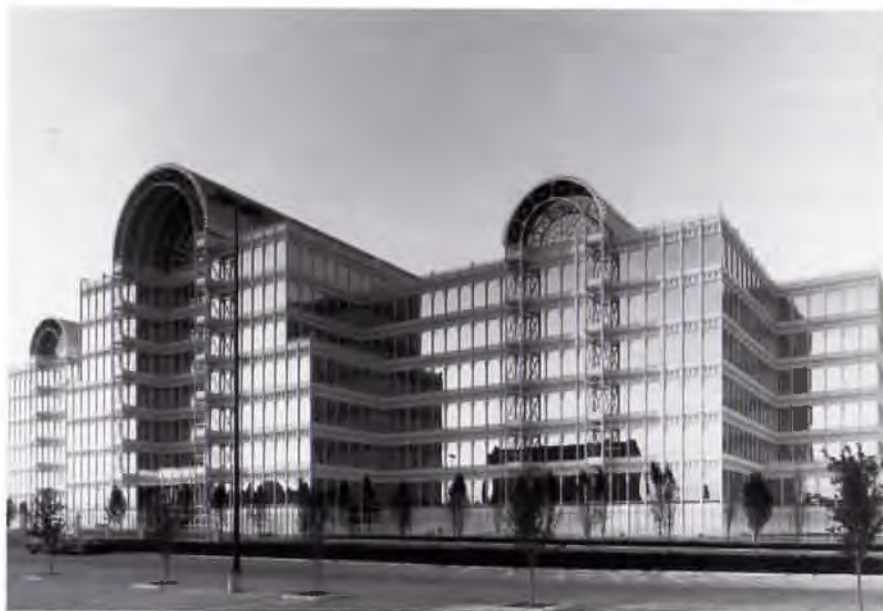
The Infomart in Dallas, designed by Martin Growald of Fort Worth, uses recycled aluminum and reflective glass to echo the imagery of Joseph Paxton's 1851 Crystal Palace in London. The nostalgic exterior wraps around a conventional concrete building housing showrooms for advanced technology.
