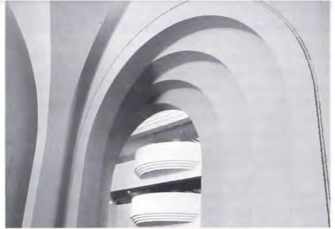
Groined roof of bar with "sliding arches" and balconies beyond.
