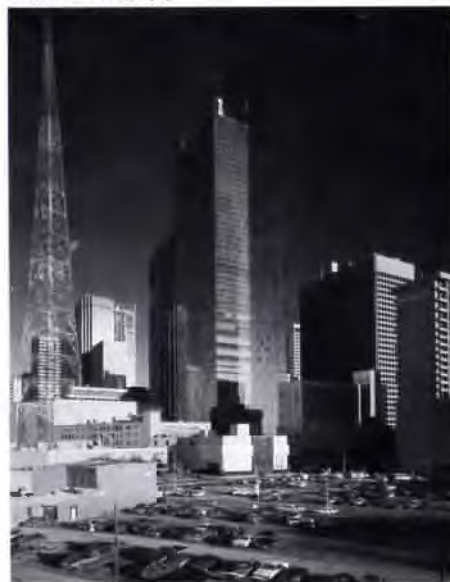
Renaissance Tower, in Dallas, is the 1975 Interfirst II Building by Harwood K. Smith and Partners, which is being re-skinned by Skidmore, Owings & Merrill of Houston.
