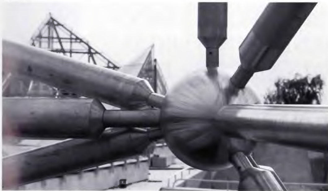
LEFT: A detail of the complex space frame over the palm house; its structure was generated by computer. BOTTOM: Section from entrance to palm house.
