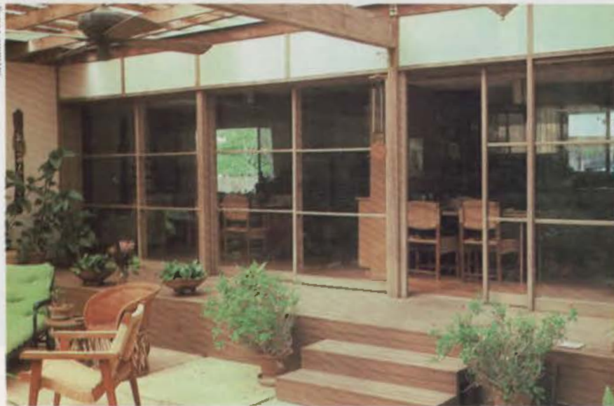
Ryan "wanted something more open." He matched an investigative, pragmatic approach to economical materials and respect for the demands of climate. TOP: The Embleton House, in Austin, shows the quality of detailing achieved by overseeing construction. CENTER LEFT: The Revere Copper House's innovative roof-cooling pond; CENTER RIGHT: Dunwoody House interior; ABOVE: The low-maintenance Seagle House, interior courtyard; OPPOSITE PAGE: Scherr House, courtyard.
