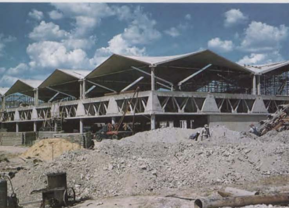
Nearly all of the Semiconductor Building's architectural components were innovative. TOP RIGHT: Concrete tetrapod truss system being mounted on the interstitial floor preceded a similar use by Kahn at the Salk Institute. TOP LEFT: Top floor is roofed with concrete hyperbolic paraboloids that permit long-spanning 63-foot-square bays. ABOVE: By 1958 the building's form began to take shape. In order to give the Semiconductor Building soaring spaces for assembling computer components, Ford reversed the traditional order of floors and placed offices and laboratories on ground level, with the manufacturing plant on the top floor above the trussed service spaces; RIGHT: Pearl Grey Georgia Marble is attached with a then-new x-shaped hanger.
