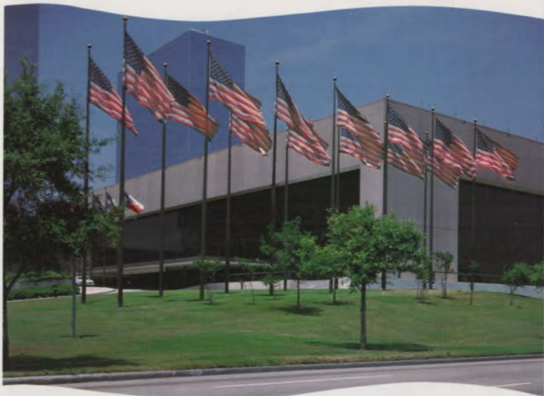
The Summit, Houston, Texas, installed, 1974.
