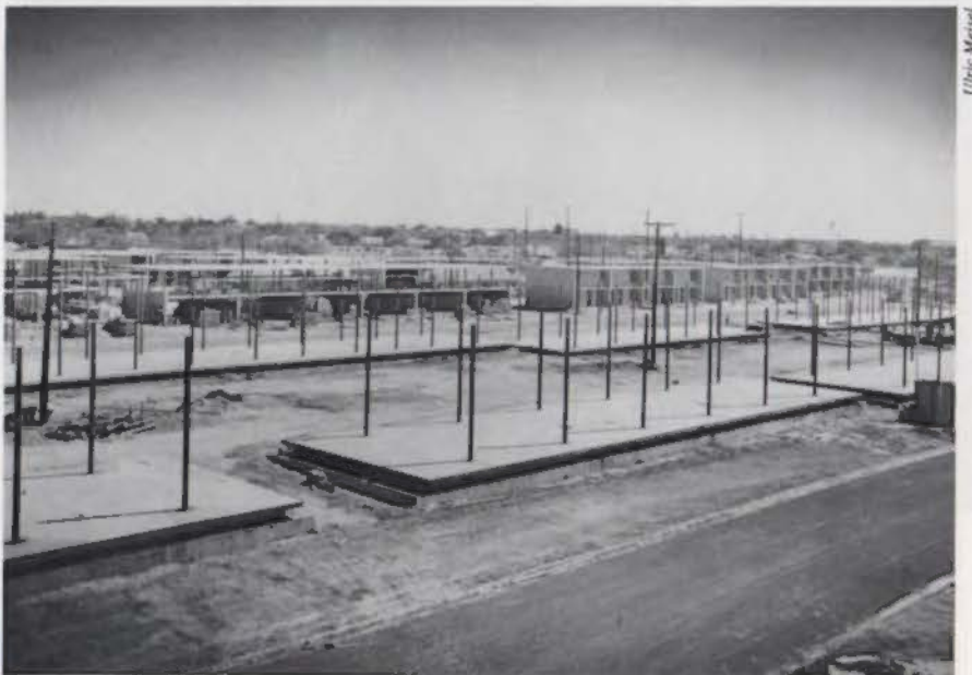
TOP: O'Neil Ford's pioneering use of lift slab began with tests conducted at Trinity University's Esser Ranch facility in 1949. A reinforced concrete slab was poured in place and then lifted hydraulically to a desired level on permanent structural steel piers. ABOVE: Ford, Powell & Carson went on to use the system extensively in Texas throughout the 1950s.
