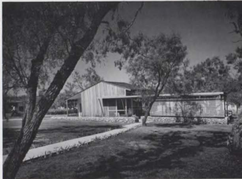
The Modernist penchant for highlighting structure found in Ryan a talented practitioner. TOP: The ethereal Lucy Dunwoody House, which Architectural Forum called "almost a diagrammatic expression of stresses." LEFT: the Sacks House was built in 1952. ABOVE: The Lohse House, 1948-1950, combines natural and industrial materials.
