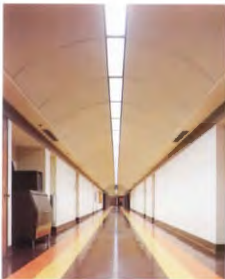
Renovated ceiling with factory-curved panels.
