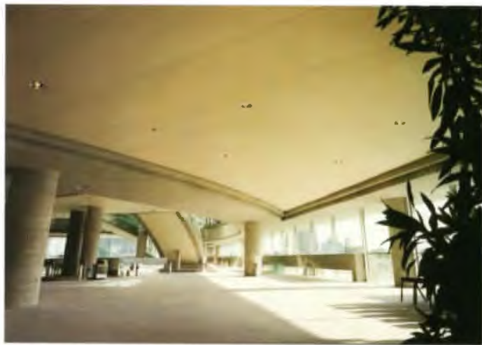
Lobby ceiling in triangular quadrants. Panels in different sizes carry curve on one edge.
