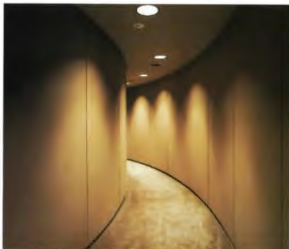
Wall panels in auditorium entrance have top and side edges bullnosed with 1/2" radius.
