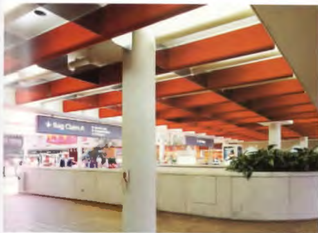
Airport baffles are 6" thick, hollow frame construction, with radius bottom edge.
