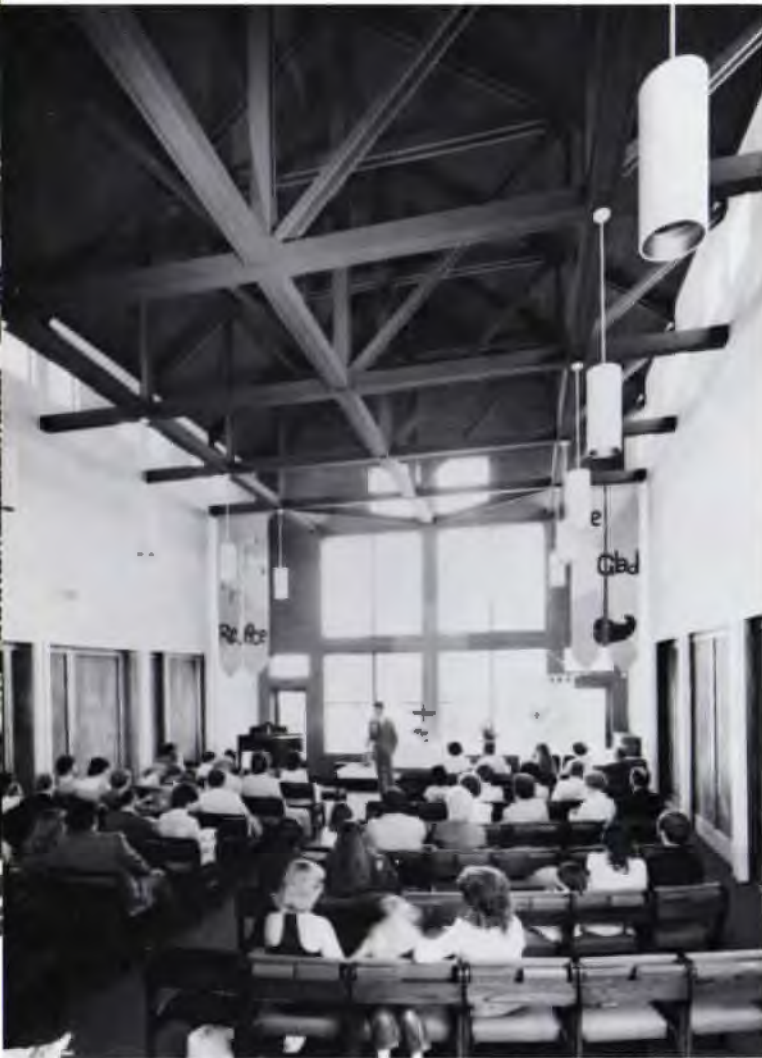
Simple, straightforward space, enlivened by a lacy network of prefabricated trusses, will serve as a parish hall after a permanent sanctuary is built.
