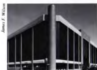
FROM TOP: Our Saviour Lutheran, Church of the Epiphany, St. Andrew's Presbyterian, Clear Lake Presbyterian, St. Barnabus Episcopal and, the epitome of "practical spirituality," First Baptist Church parking garage, Dallas (Hatfield Halcomb Architects).
