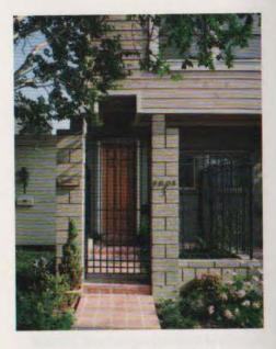
raised landing of the stair, required to satisfy the building code requirement of no continuous vertical run more than 12<sup>1</sup>/<sub>2</sub> feet, allowed the creation of a recess above the front door in the soffit of the second-floor overhang—possibly to be read as an allusion to a ceremonial entry portal.
