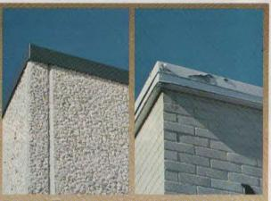
Examples of building gravel stops with factory-applied Kynar 500 (left) and field-painted finish (right).
