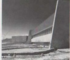
Vertical fins and deep recesses reduce heat load.
