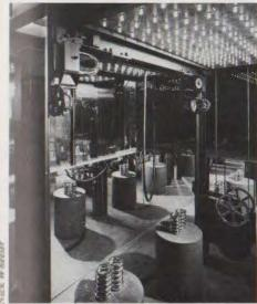
Underside of elevator and mirror-clad pit; chrome springs and gear wheels.
