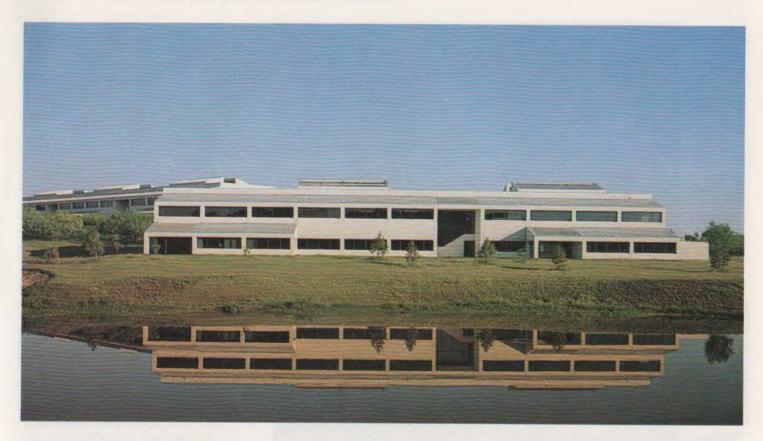
perimeter bays hung like saddlebags from each side of the box. Their sloping shed roofs are of standing-seam metal, with cedar trellises over glass areas where the glazing extends from floor to ceiling. The sloping roof motif is repeated on the flat roof of the box by "sheds" covering the conventional mechanical equipment, to shade as well as hide it when a highrise goes up nearby. Recessed windows are of tinted glass, and the exterior finish is stucco.
