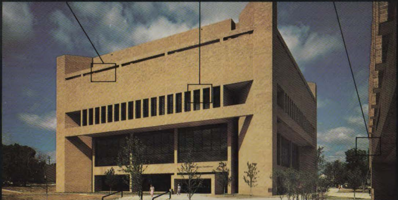
Collin County Courthouse and Jail, McKinney, Texas Owner: Collin County, Texas Architect: Jarvis Putty Jarvis, Inc., Dallas, Texas Structural Engineer: Datum Structures Engineering, Inc., Dallas, Texas Masonry and General Contractor: Howard U. Freeman Incorporated, Irving, Texas
