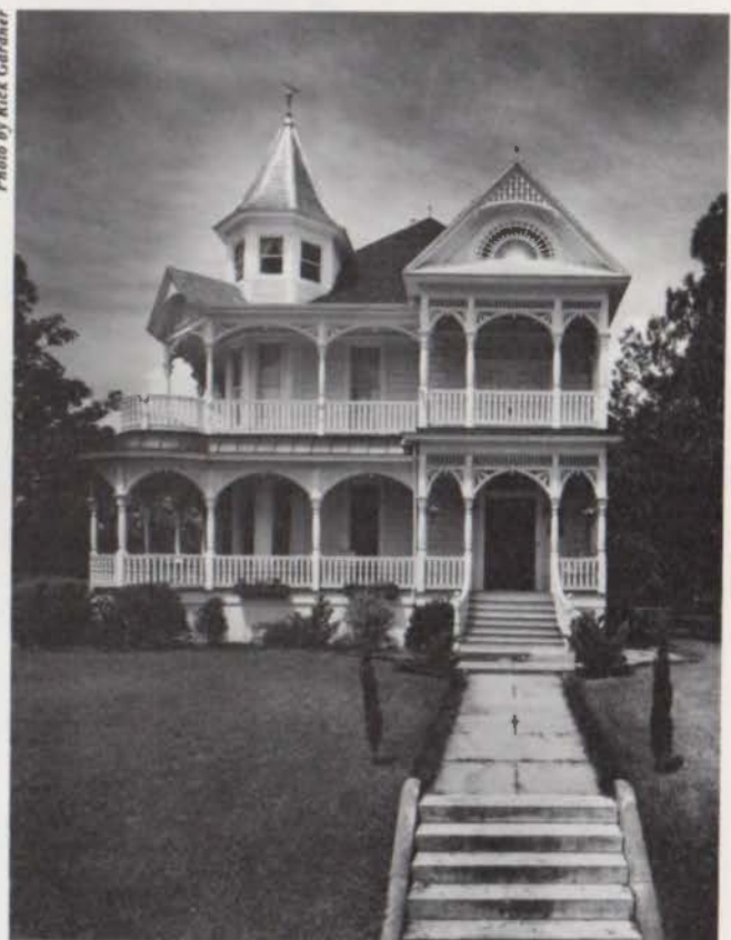
Wood House, Brenham, 1897.
