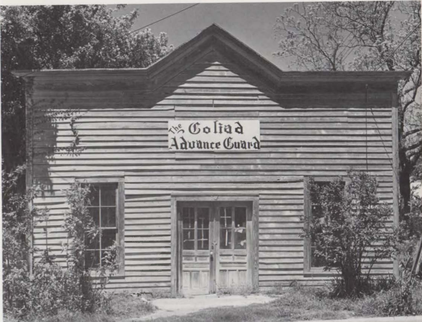
Former home of Texas' second oldest newspaper. Original structure established circa 1850.
