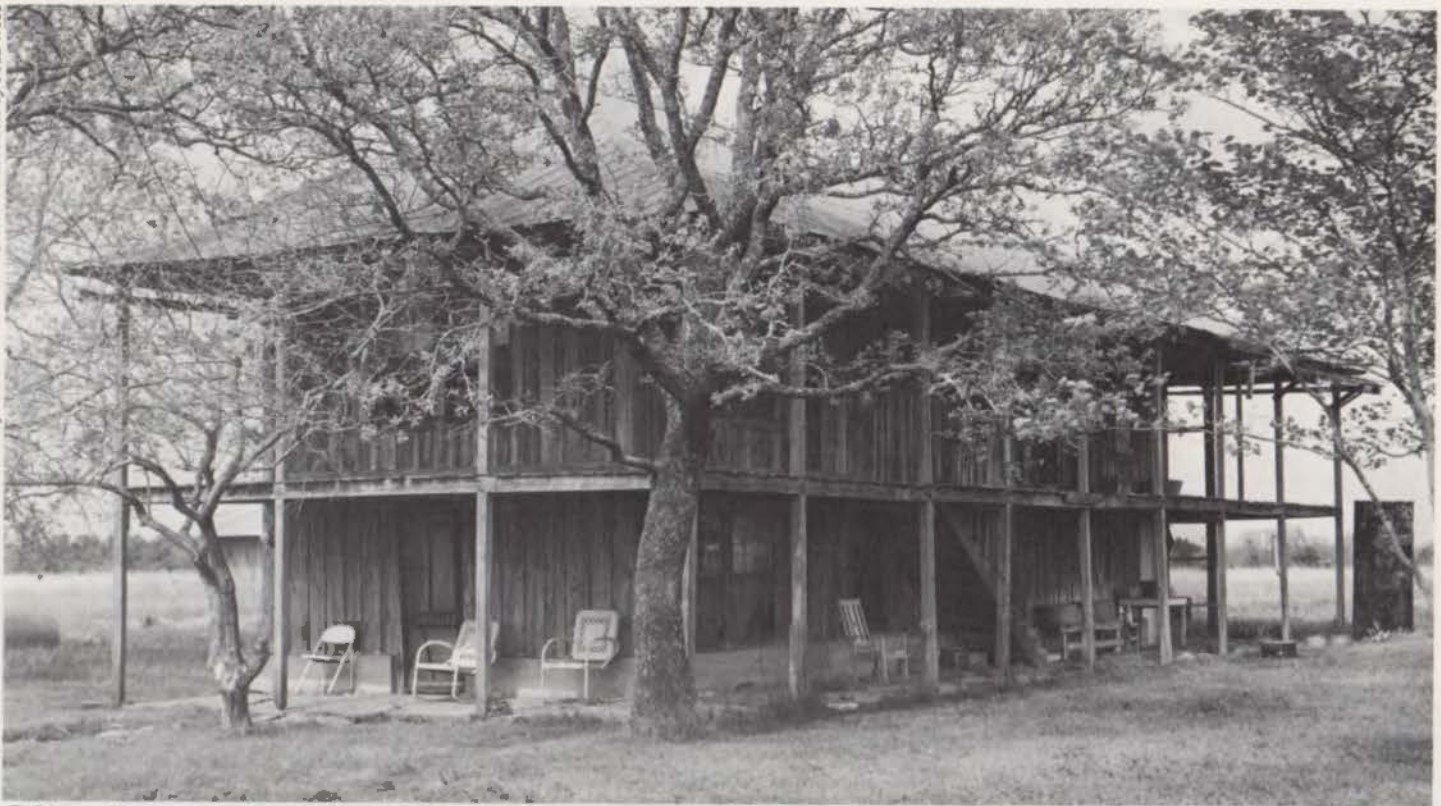
Cabiness House, near Huntsville, 1915.
