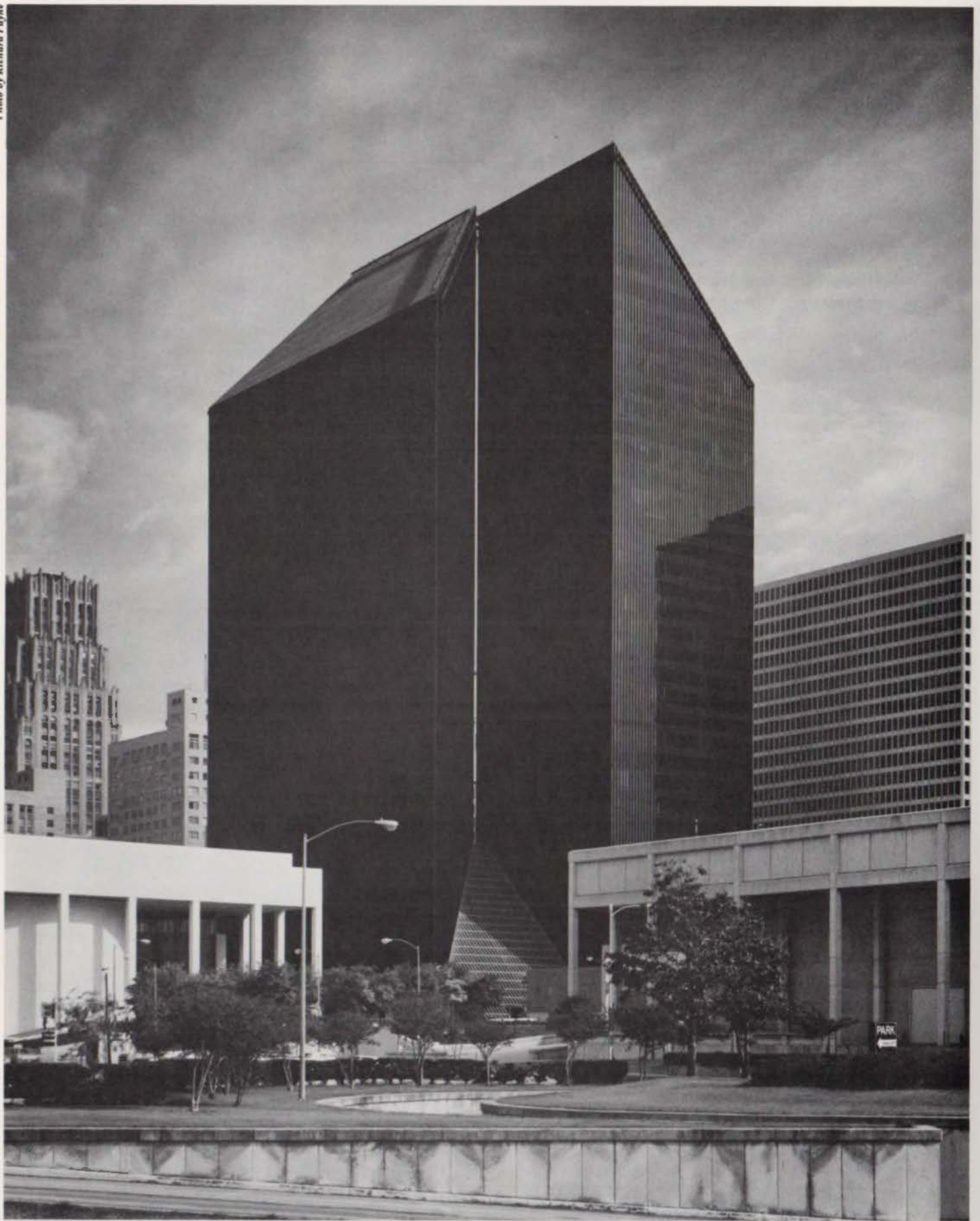
Pennzoil Place, Houston, 1976. Johnson|Burgee, architects. S. I. Morris Associates, associate architects.
