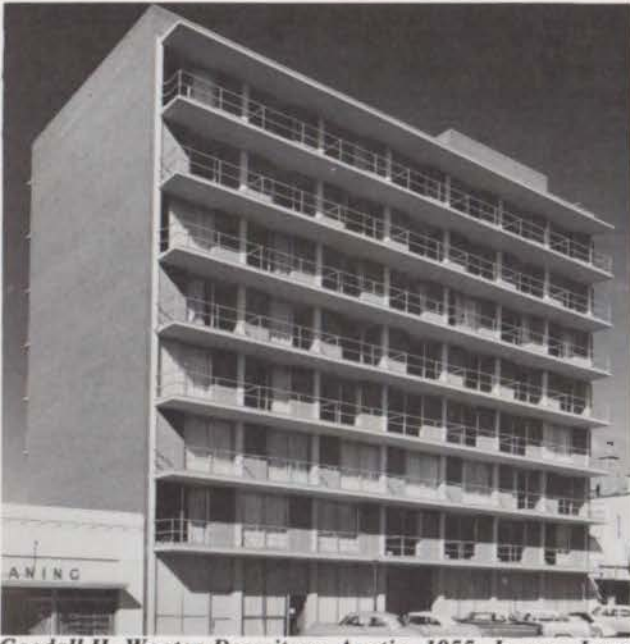
Goodall H. Wooten Dormitory, Austin, 1955. Jessen, Jessen, Millhouse & Greeven, architects.
