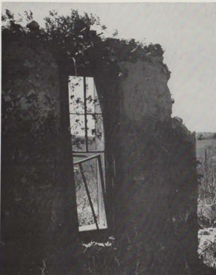
These walls, the remains of a residence at Kimball, were constructed of "Tabby" — a type of concrete used extensively during the Nineteenth Century.
