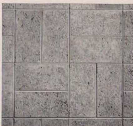
BASKET WEAVE. Laying 8x8x16-in. block in pairs, two vertically and two horizontally, and tooling all the joints results in this woven pattern for interior non-bearing walls.
