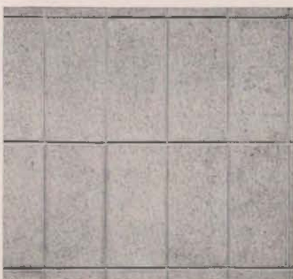
VERTICAL STACKING. Like horizontal stacking except that the block are laid on end. This unusual pattern creates illusion of greater height for interior non-bearing walls.
