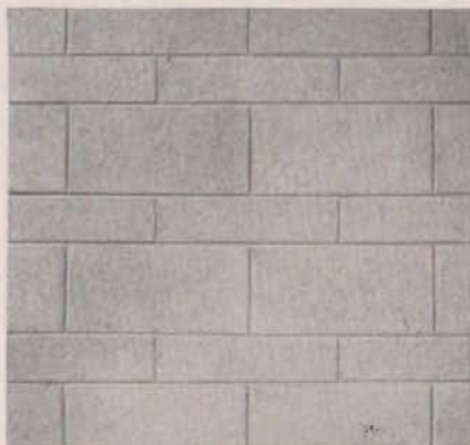
ALTERNATE RUNNING BOND. Alternate 8-in. and 4-in. courses, tooling all joints, to produce this charming effect. For variation use 4-in. units every third or fourth course.
