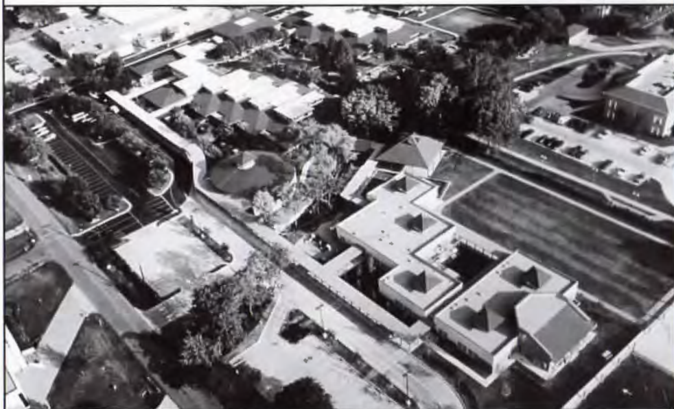
THE FOCAL POINT ON ST. ALCUIN'S CAMPUS IS THE ROUND ROOF CLAD WITH BERRIDGE TAPERED HIGH SEAM TEE-PANELS. BERRIDGE'S CEE-LOCK STANDING SEAM SYSTEM WAS USED FOR STRAIGHT PANELS ON OTHER ROOF AREAS.
