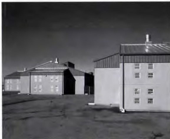
Right and bottom far right: Housing buildings were constructed with factory-cast concrete cell units transported to the site.
