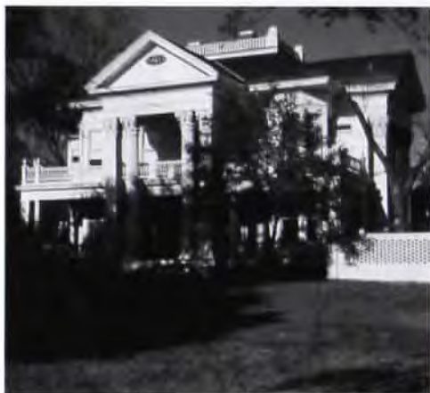
Above: 600 E. 29th Street, a Greek Revival-style house from 1910, finds protection under Bryan's new historic preservation guidelines.
