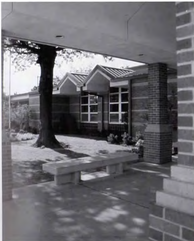
Left: Canopies covering benches highlight the school's entrance
