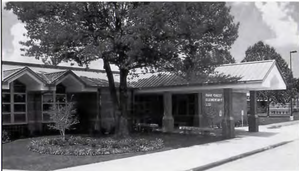
BERRIDGE TEE-PANEL STANDING SEAM ROOF PANELS, FINISHED IN KYNAR 500® "HEMLOCK GREEN", SERVE AS A UNIFYING ELEMENT TO LEND CONTINUITY BETWEEN EXISTING AND NEW SPACE IN THE RENOVATION OF PARK CREST ELEMENTARY SCHOOL, GARLAND ISD.
