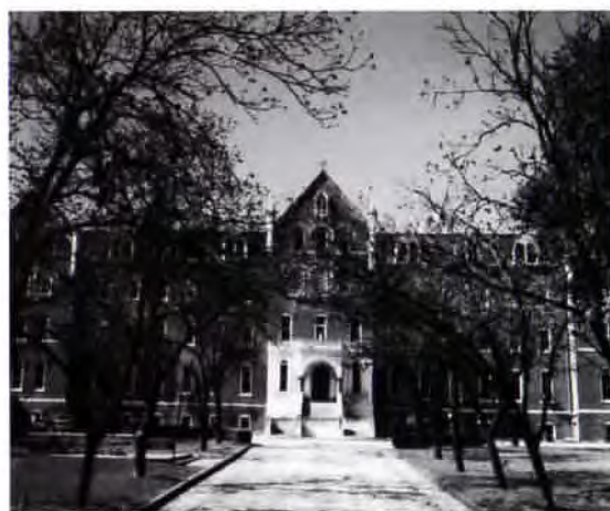
Incarnate Word Mother House, original building (see p. 32 for Jones & Kell's award-winning project)
