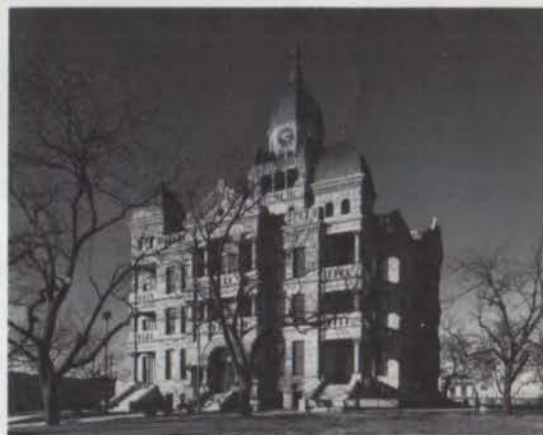
Above: New central air conditioning made it possible to remove numerous window units from the courthouse's Richardsonian Romanesque facade.
