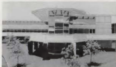
Conoco Building, 1985, by Roche Dinkeloo
