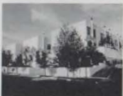
Travis Street Condominiums 30
